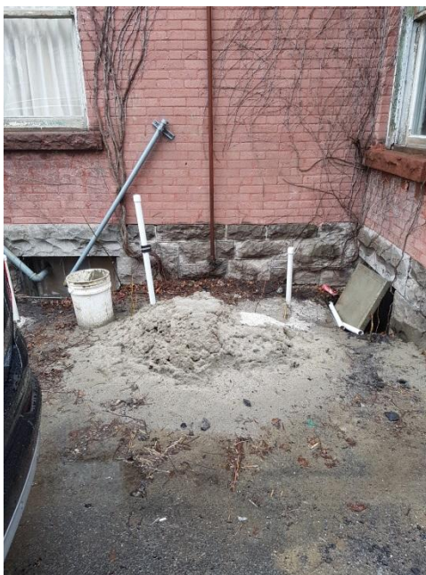
Photograph 32. 22 Hawthorne Ave – view of northeast wall from 24 Hawthorne Ave asphalt driveway; possible location of former oil tank (excavation cuttings and monitoring wells present)
