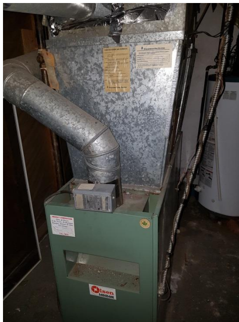
Photograph 16. Interior of 24 Hawthorne Ave – natural gas-fired furnace in basement
