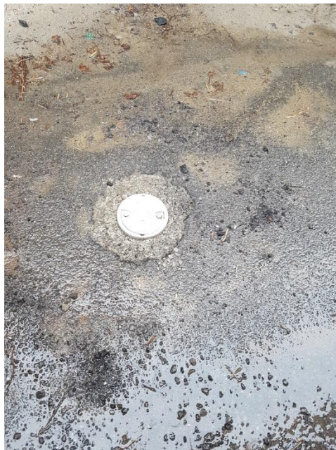
Photograph 34. 22 Hawthorne Ave – view of flushmount monitoring well installed along 22/24 Hawthorne Ave property line, in asphalt driveway
