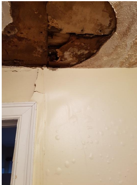
Photograph 12. Interior of 24 Hawthorne Ave – second floor water damage
