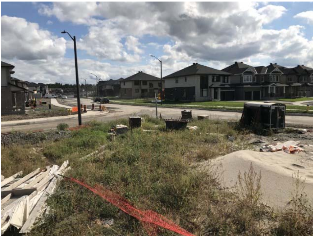
Photo 8: View of southwest corner of Site, some construction materials present on Site, facing southwest.
