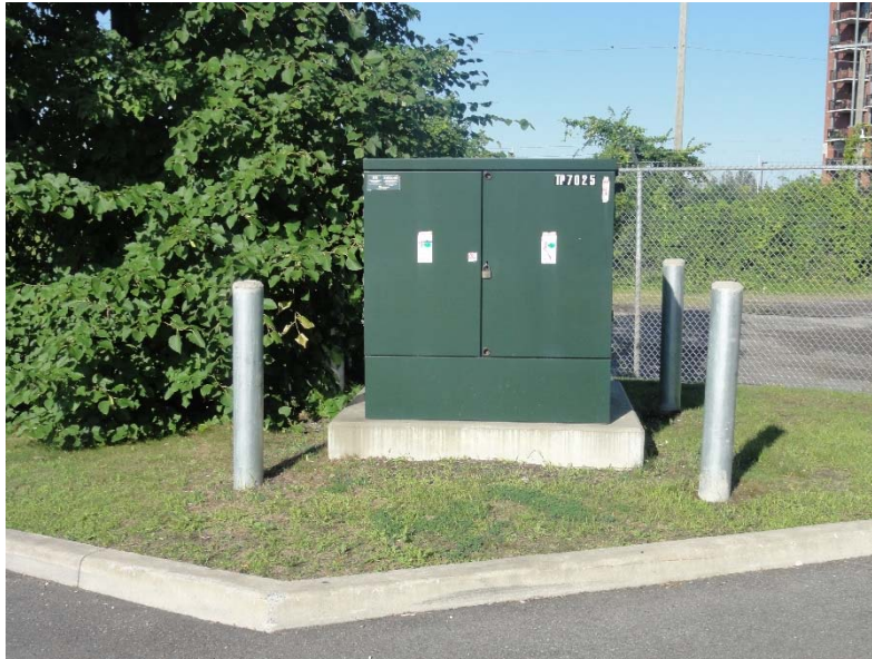
Photo 9 – View of the concrete pad mounted transformer on the northwest portion of the Site.
