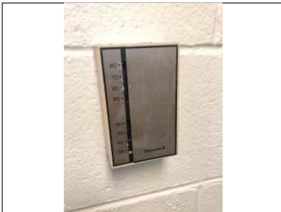
Photograph 20: View of thermostat containing mercury
