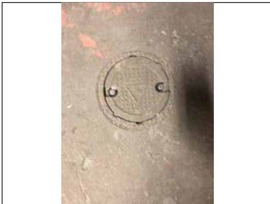
Photograph 19: View of interior monitoring well
