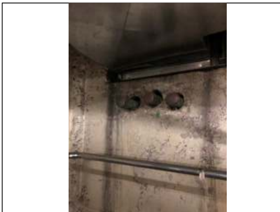
Photograph 18: View of decommissioned fuel oil supply lines
