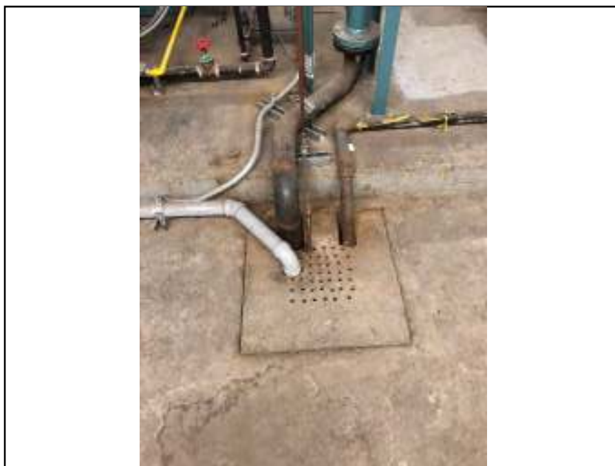
Photograph 20: View of floor drain in boiler room
