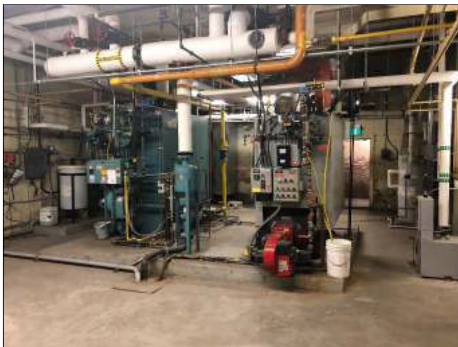
Photograph 16: : View of natural gas fired boilers
