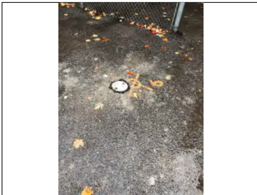
Photograph 11: View of exterior geotechnical monitoring well
