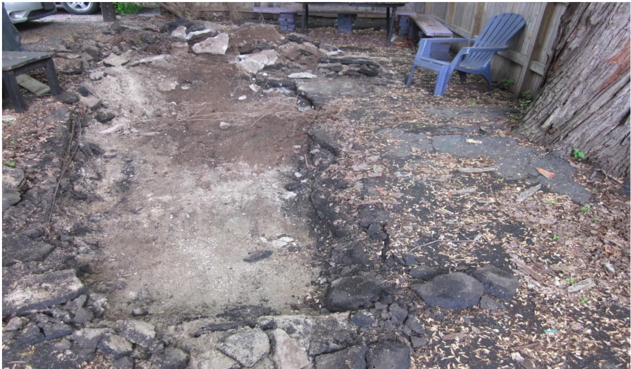
Picture 4. Layers of asphalt removed prior to root investigation of red maple shared between 419 and 423 McLeod Street. Note lack of pronounced flaring at base of tree on right. Also note soil and fine roots directly beneath asphalt layer.
