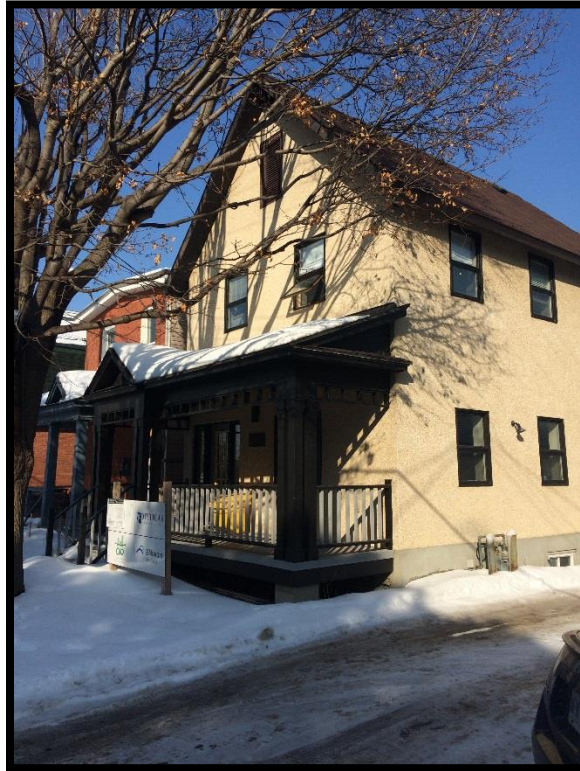
Photograph 1: View of the west building face.
