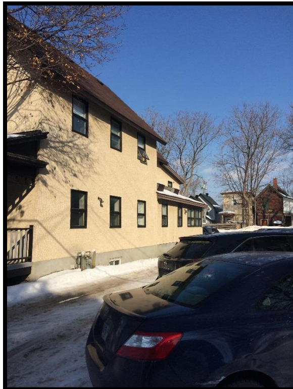
Photograph 2: View of the south building face, and parking lot.
