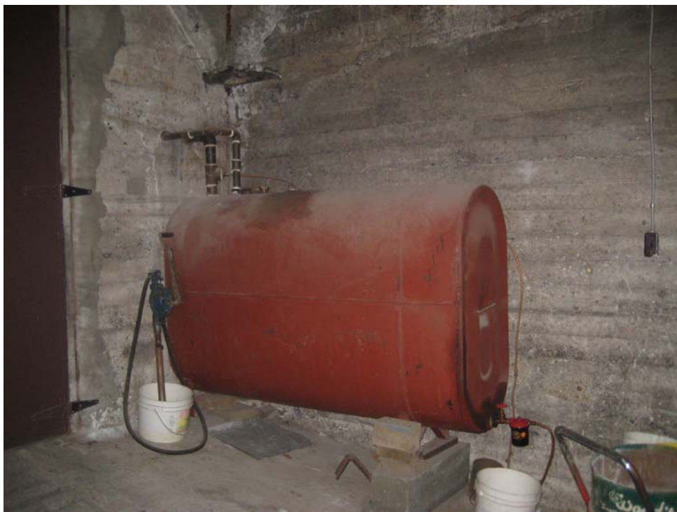
Photograph 16: View of the diesel AST located in the former coal storage room and used to fuel the backup generator.
