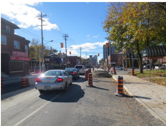
11. View of Rideau Street, facing west.
