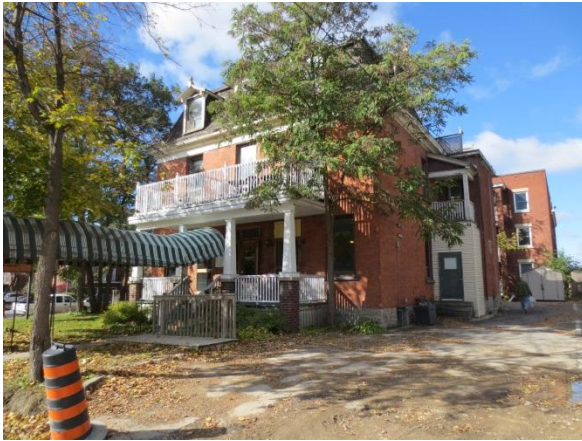
1. View of the Phase One Property, facing north.
