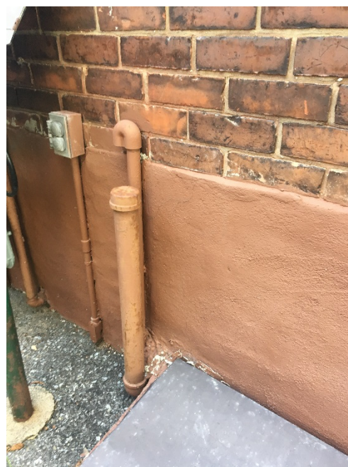
Photo 4: Fill and vent pipes for the basement AST at 130 Robinson Avenue
