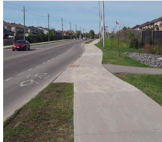
Figure 8. Fernbank Road: west towards pathway
