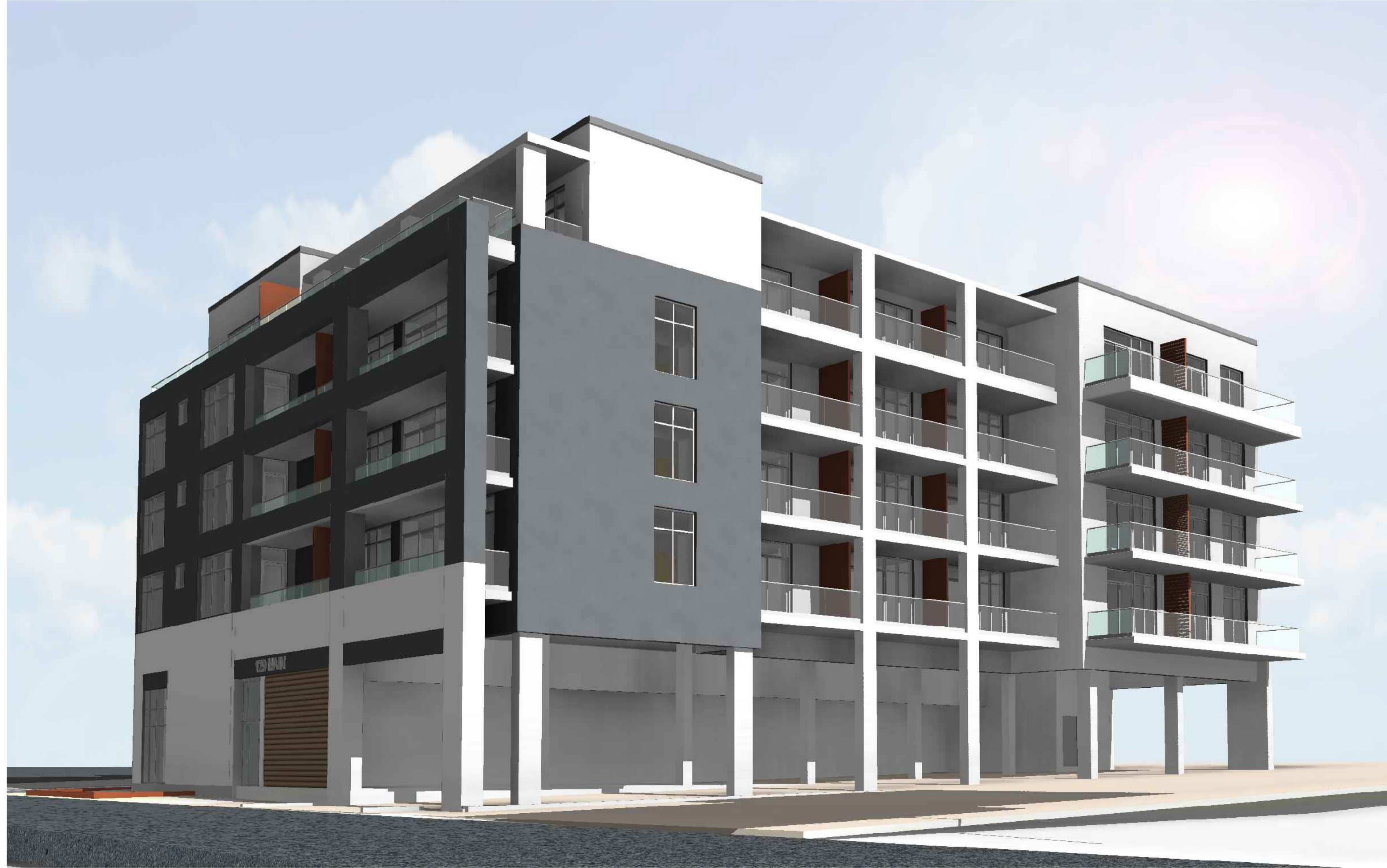
VIEW LOOKING WEST ON SPRINGHURST AVENUE
