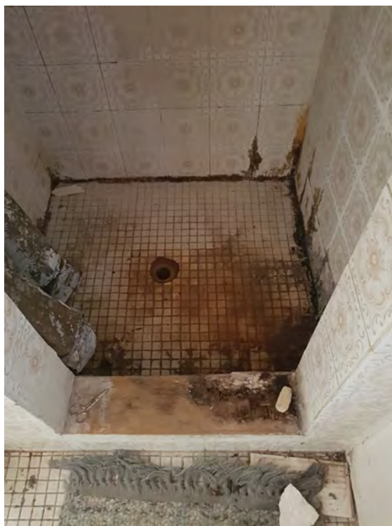
Photo 16: Basement bathroom, mould-like substances on tiles
