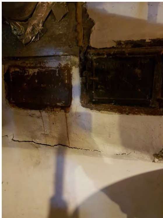
Photo 19: Basement furnace room, ash cleanout with cracks in wall
