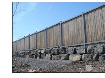
THE ABOVE IMAGE INDICATES THE PROPOSED WOODEN PRIVACY FENCE. THE FENCE IS TO BE 1.8m HIGH, PREMIA BY PRESTIGE FENCE, OR APPROVED EQUIVALENT. FENCE POSTS AND RAILS IN THIS SAMPLE IMAGE ARE GREY, BRONZE WILL BE SPECIFIED FOR THIS BLOCK TO MATCH WITH THE SURROUNDING
