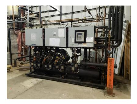
Photograph 8: View of the compressors serving the refrigeration and freezer units of the Tannis subject building.
