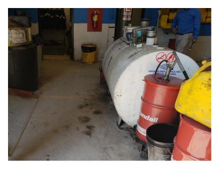
Photograph 1: Above ground used oil storage tank inside the Thermo King service bay.
