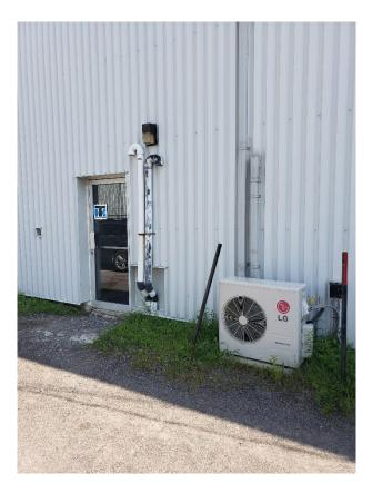
Photograph 4: View of the west facing façade of the Thermo King subject building. Air condition serves the office area and the vent pipes are presumed to serve the service bay catch basins.
