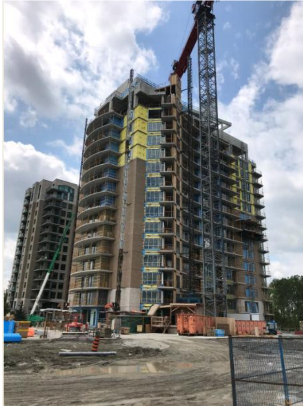
Figure 5: View of Tower 2 Under Construction
