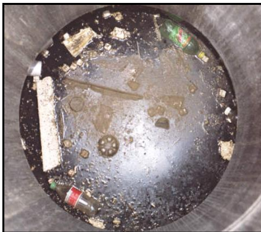
Floatable debris in the Aqua-Swirl®
