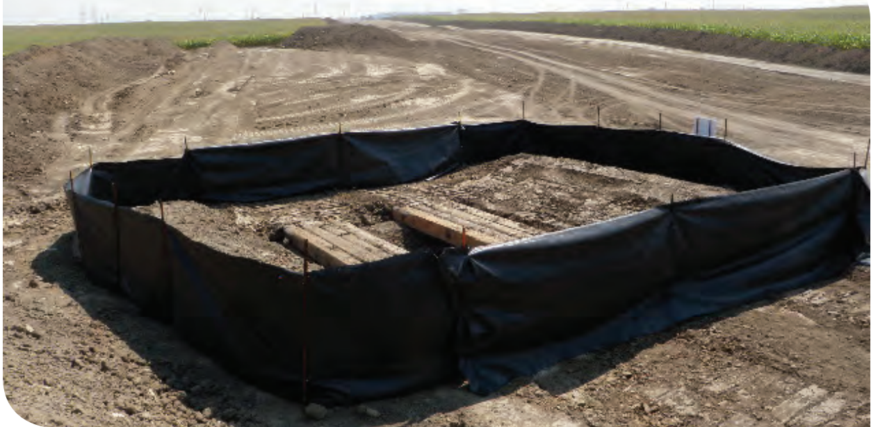
Cleaning station at construction site.
