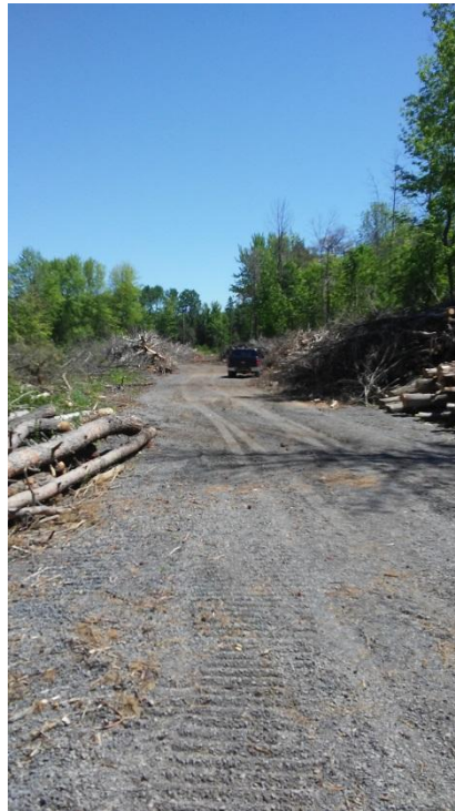
Photo 2: On-site construction laneway, view from Franktown Road
