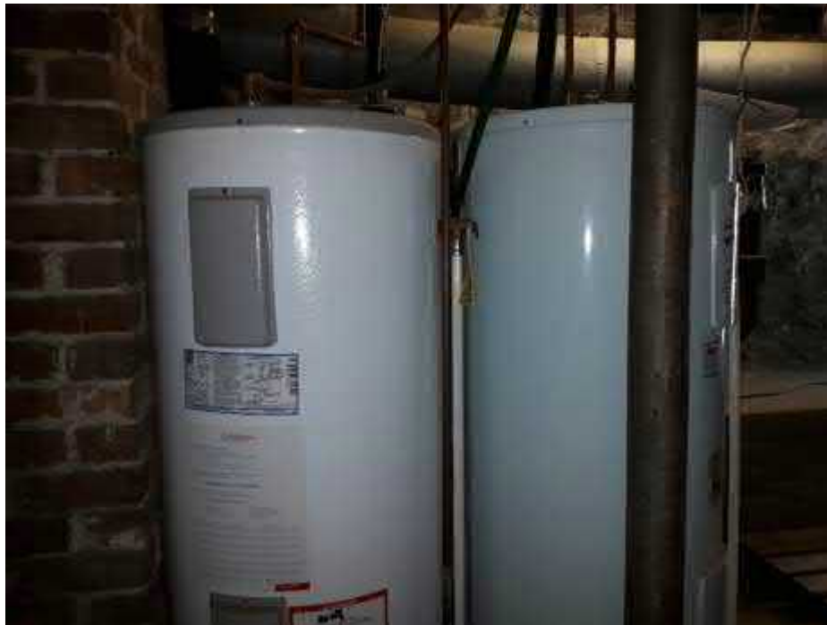
Photograph 5. Basement of residence beside furnace #2, showing hot water tanks for 2 units.
