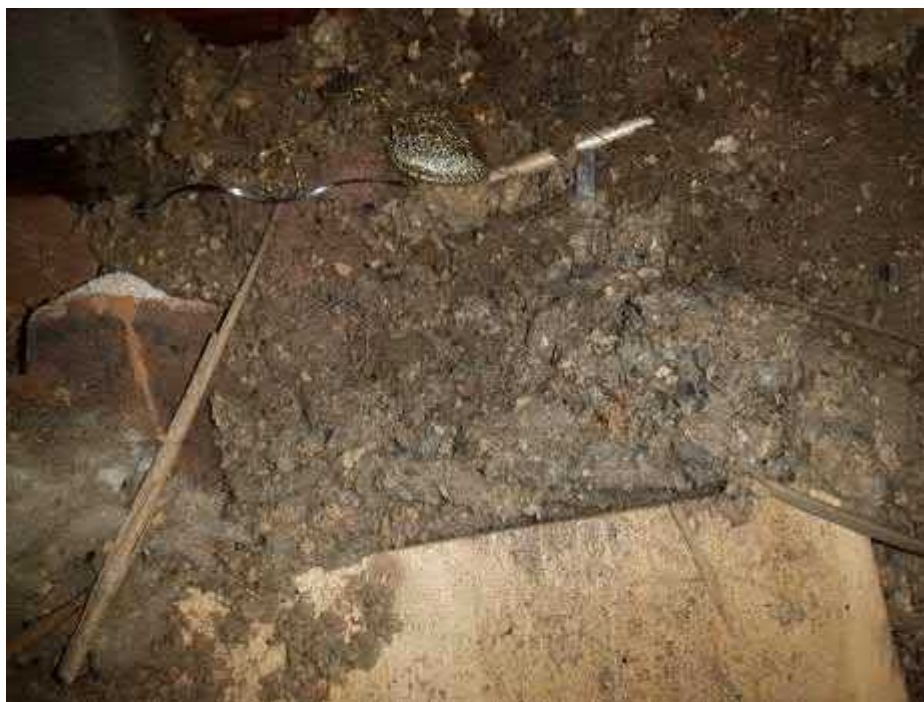
Photograph 12. Attic space of residence, a mix of insulation types present, possible vermiculite insulation
