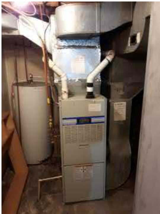
Photograph 3. Basement of residence, Furnace #1 with hot water tank and floor drain
