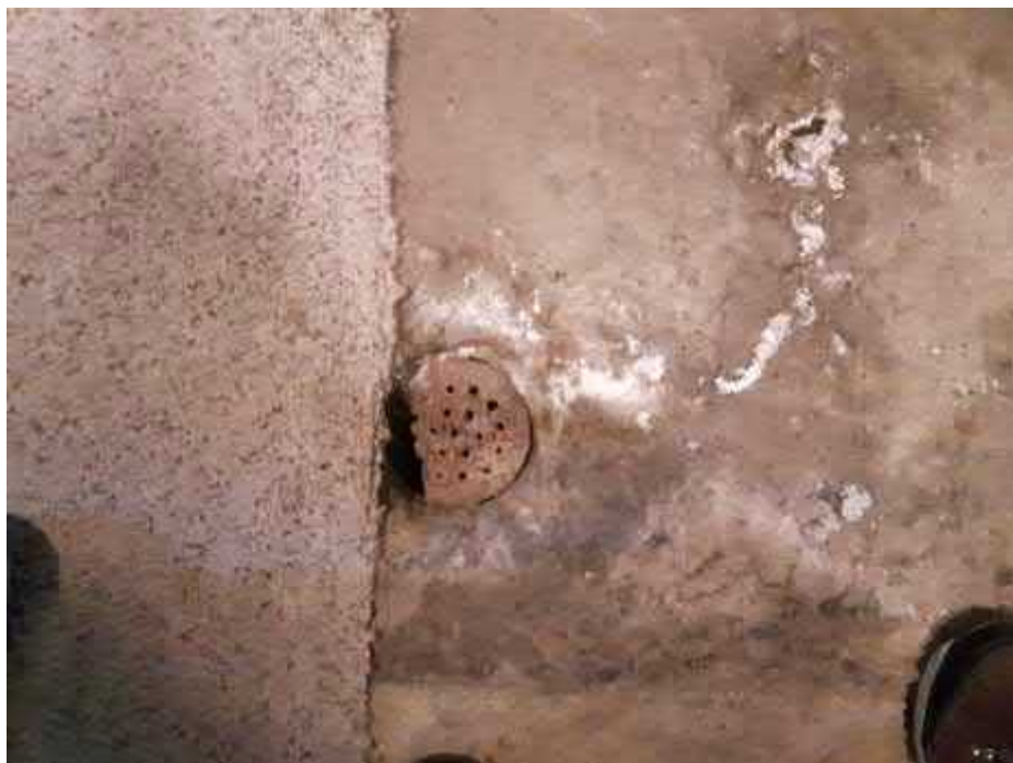
Photograph 9. Basement of residence, floor drain in proximity of Furnace #1. Slight staining, no odour
