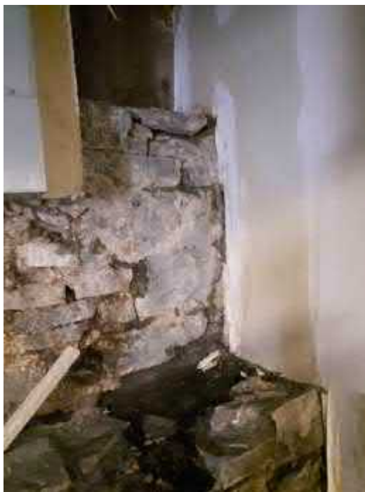
Photograph 6. Basement of residence beside furnace #2, stone foundation with extensive water damage and apparent mould
