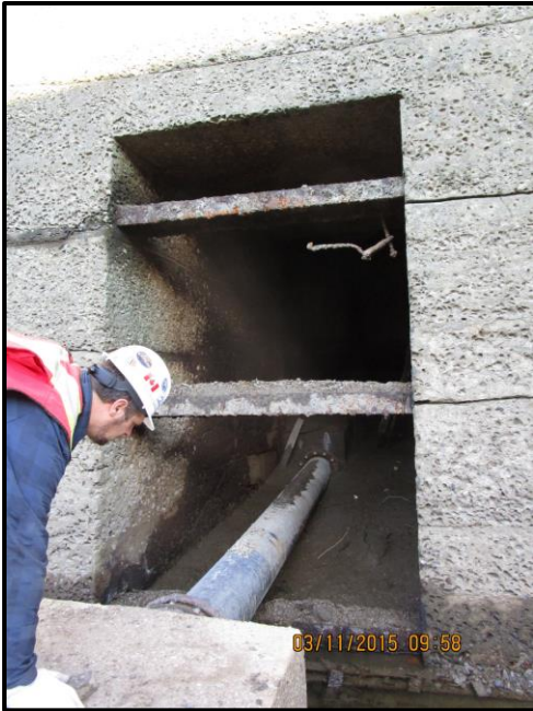
Photograph 9: Water intake in the Buchanan Channel wall. The intake is shown when the channel was dewatered in November 2015 to allow maintenance access. The water intake is normally submerged beneath the water surface.
