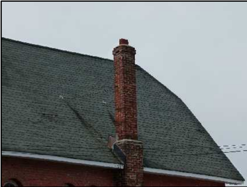
Photograph 4: 115 Echo Drive chimney (May 15, 2015). Note that a ceramic liner is evident.
