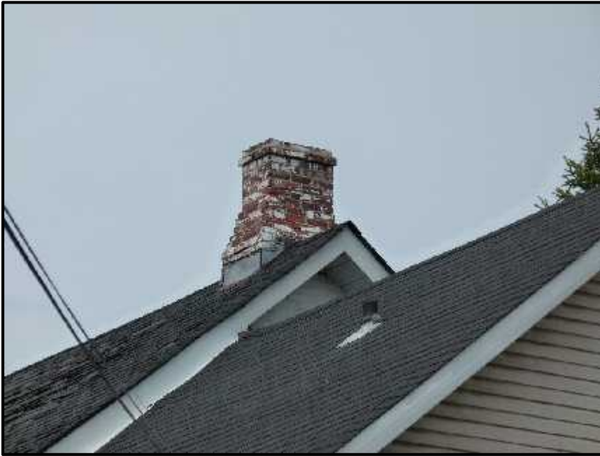
Photograph 3: 113 Echo Drive chimney (May 15, 2015). Note that no liner or cap on the chimney is evident.
