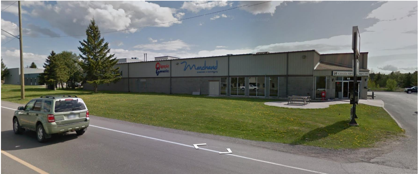
Figure 3: Streetview of existing building at 44 Iber Rd.
