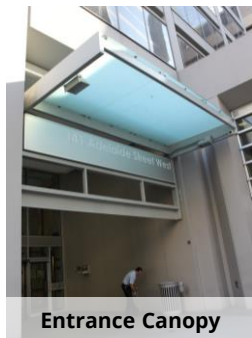
Image 7 – Examples of Wind Control Features for the Entrances along Woodroffe Ave.
