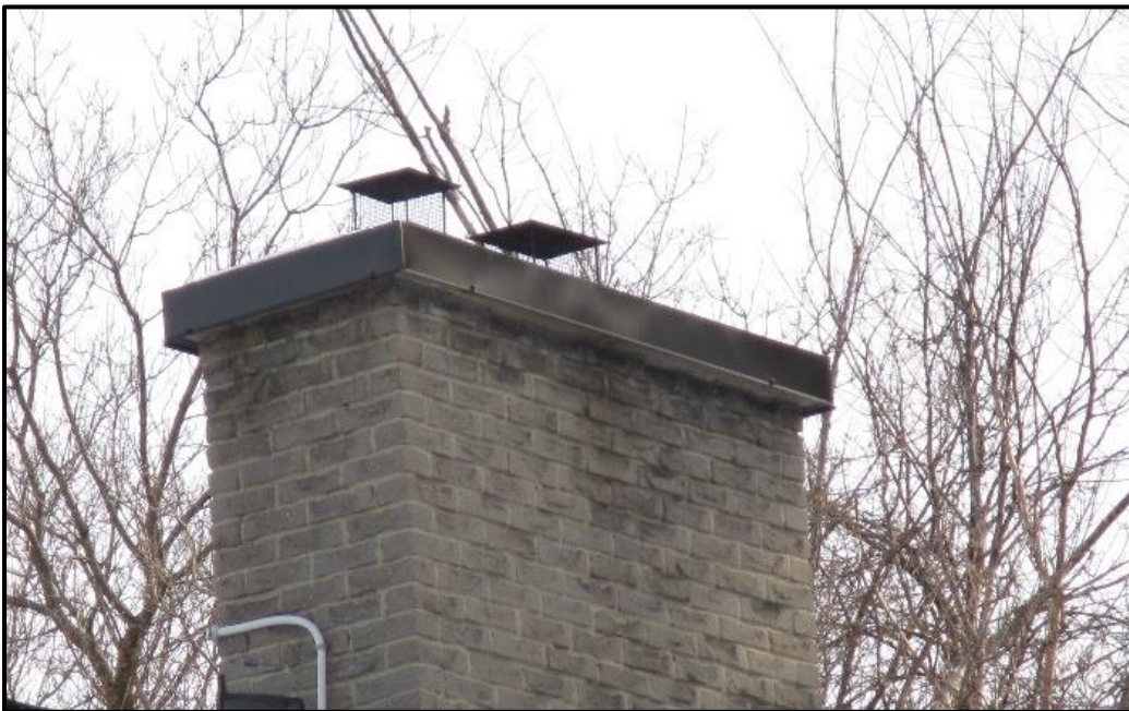
Photograph 10: Chimney at 1054 Hunt Club Road. Note wire mesh cap on chimney (February 6 th , 2017).
