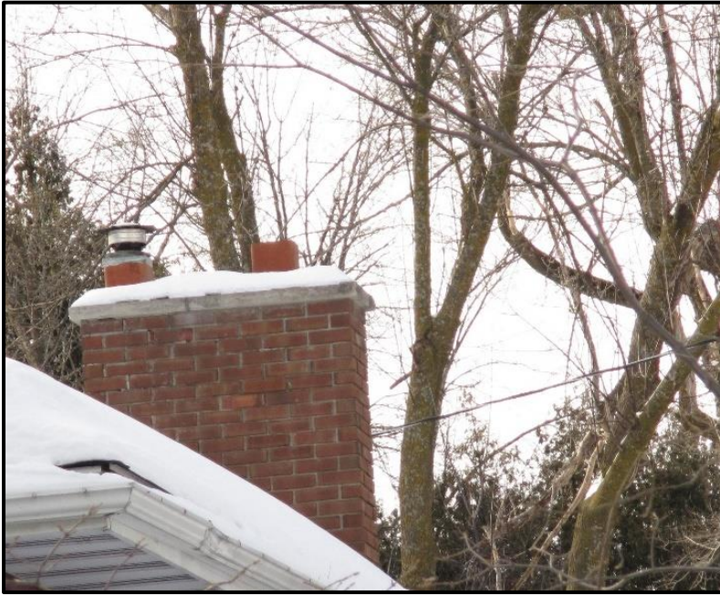
Photograph 11: Chimney at 1040 Hunt Club Road. Note metal cap and ceramic liner (February 6 th , 2017).
