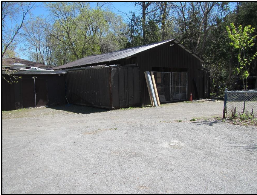
Photograph 7: Storage shed at 1038 Hunt Club Road. Note painted metal siding on wooden frame (May 15 th , 2017).
