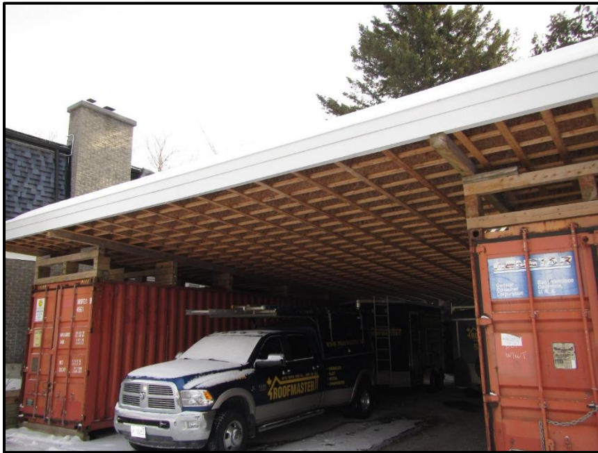
Photograph 3: Temporary covered work area at 1054 Hunt Club Road. Note wooden lattice roof on shipping containers (February 6 th , 2017).
