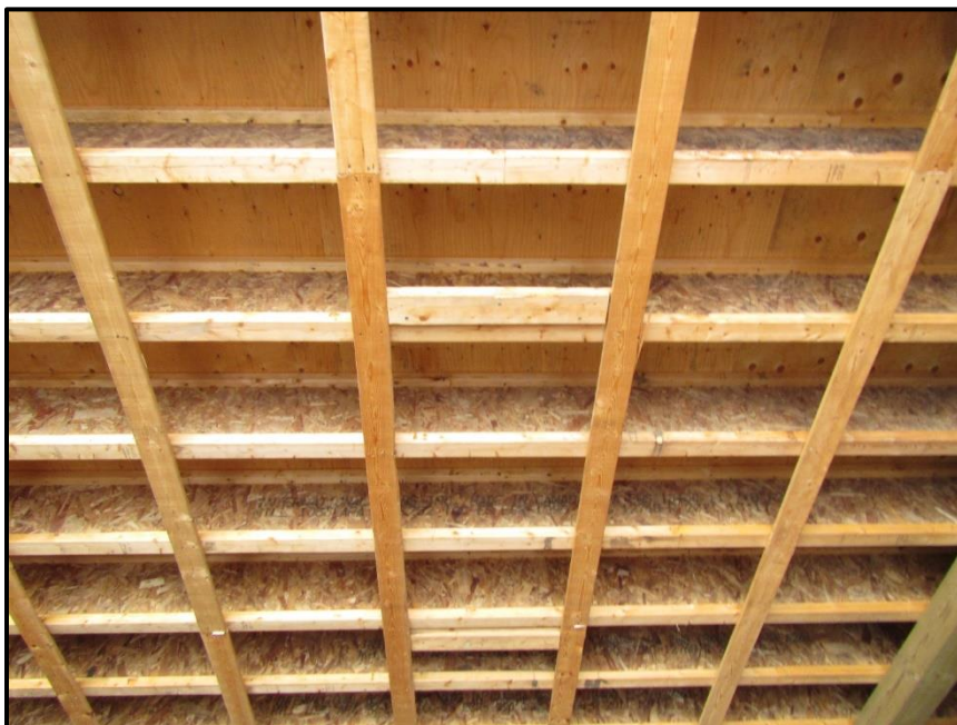
Photograph 4: Roof of temporary covered work area at 1054 Hunt Club Road. Note wooden lattice roof on shipping containers (May 15 th , 2017).
