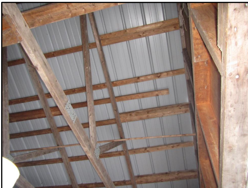
Photograph 8: Interior of storage shed at 1038 Hunt Club Road. Note painted metal siding on wooden frame (May 15 th , 2017).
