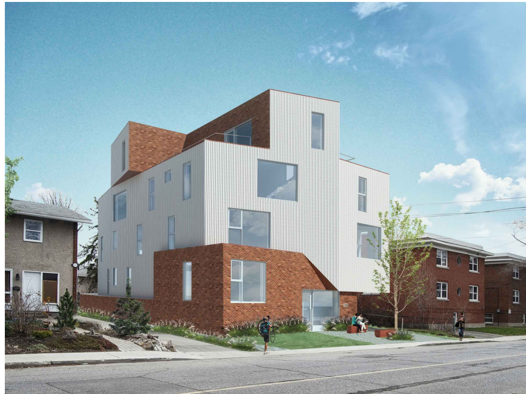
Street view from N-W
