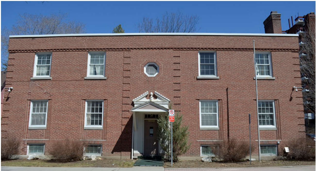
West (Main) Elevation at Cobourg Street.
