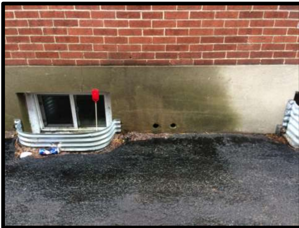
Photograph 3: View of former vent/fill pipe holes in foundation. Moisture from meltwater and rain dripping from the roof. No sheen was observed or petroleum odours were identified in the vicinity of the holes.
