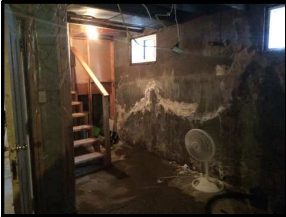
Photograph 1: View of former aboveground storage tank area in unfinished portion of the basement. Moisture on walls and floor are from weeping foundation. No oil staining or odour was observed.
