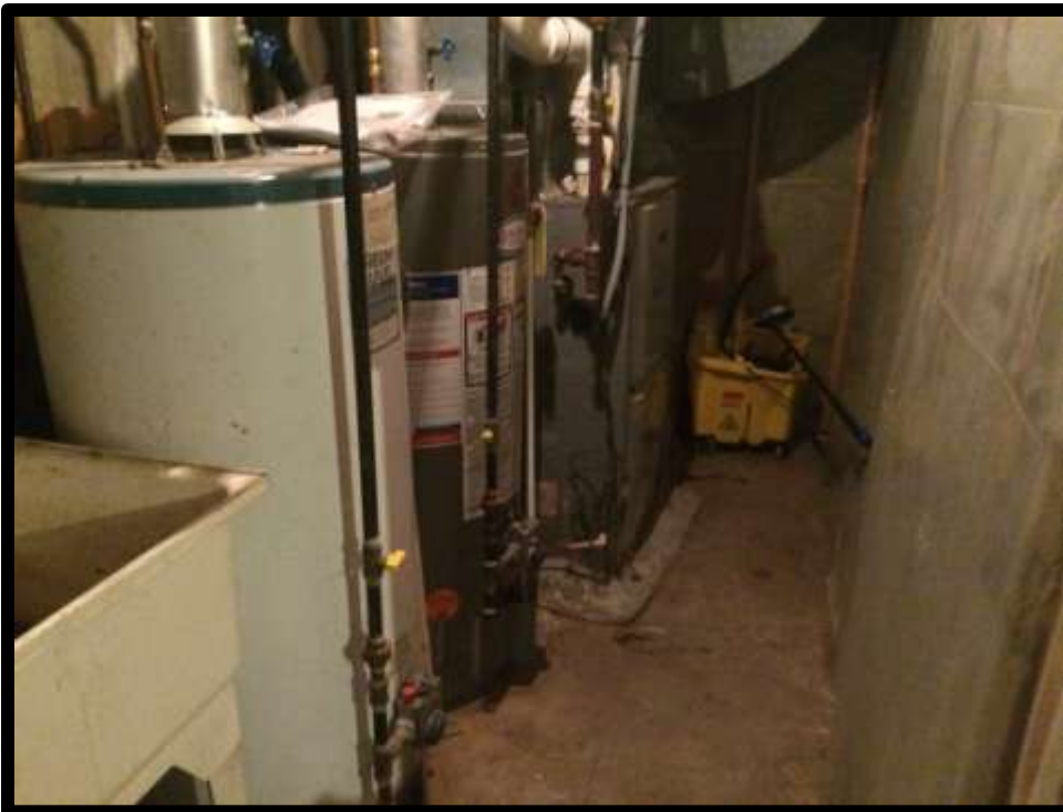
Photograph 2: View of furnace, water heaters and remnant fuel line from historical oil system.
