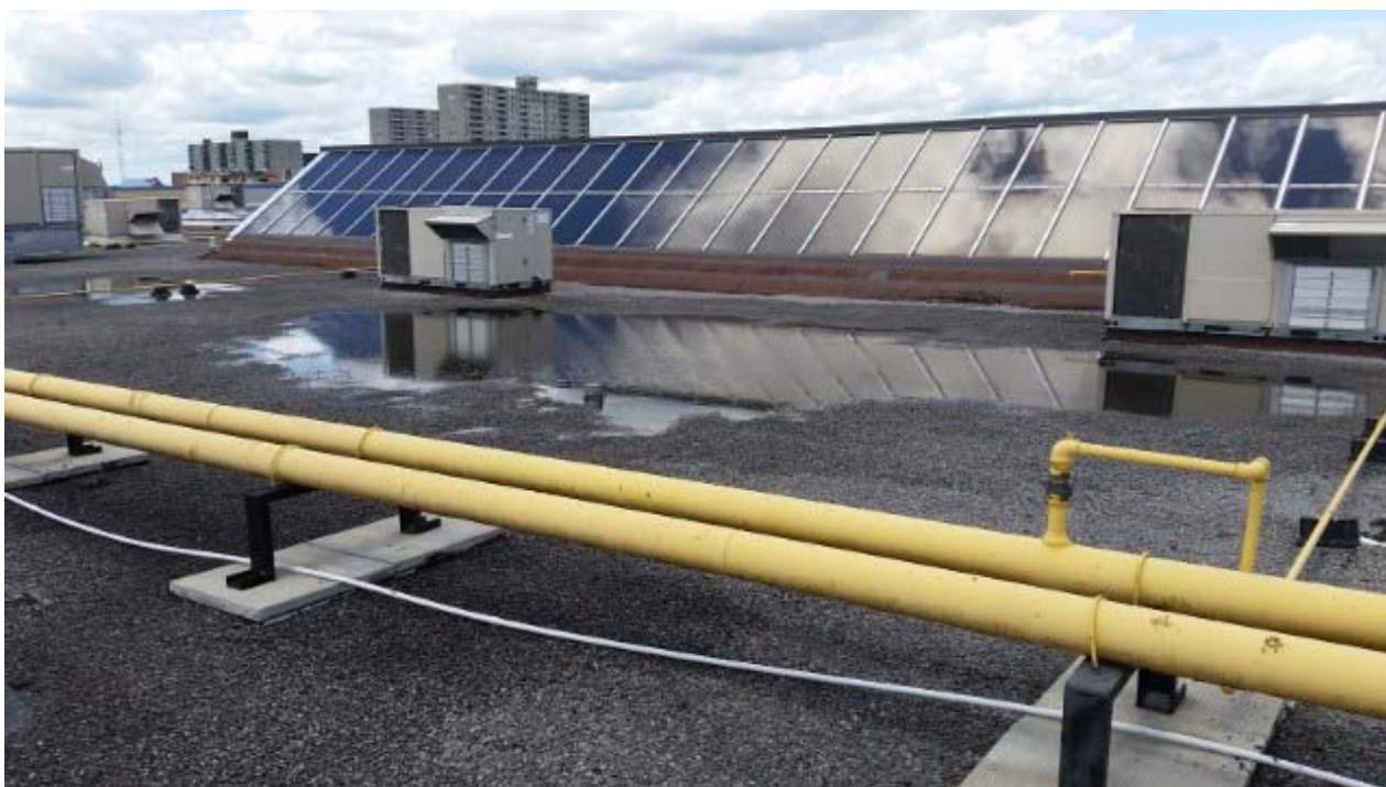
Photo 12: Pooling water was noted in several locations on the roof.
