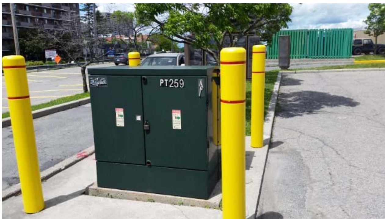
Photo 20: Pad mounted transformer north of the Wendy's building in the parking lot.
