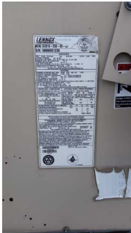
Photo 14: Several of the AC units on the roof contained R22 which is listed as an ODS.
