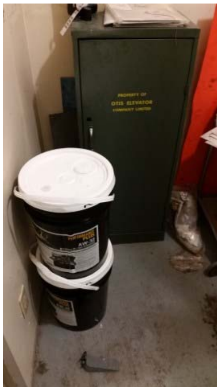
Photo 9: Hydraulic oil for refilling the hydraulic elevator AST.
