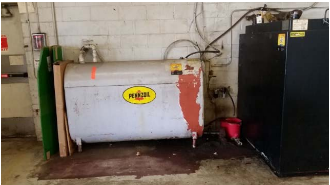
Photo 4: Bulk storage AST in the former Walmart auto service bays. Staining noted.
