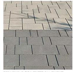
PERMEABLE CONCRETE PAVEMENT FOR WALKWAYS (POPS SIDEWALK LEVEL)
