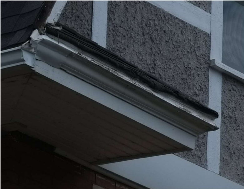
Fig. 10 and Fig. 11: Crown mouldings have deteriorated pass point of repair. Aluminum caps on the end of the crown mouldings are visible in both photos
