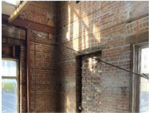
Figure 41: Steel cable at northwest corner
