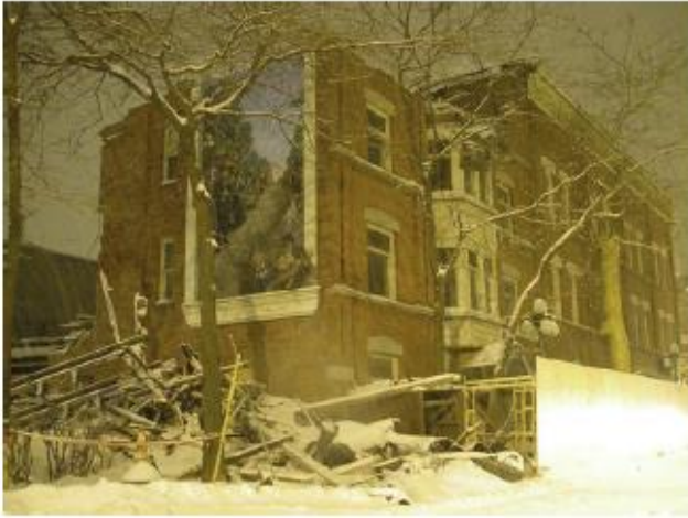
Figure 3: Somerset House after 2007 partial demolition
