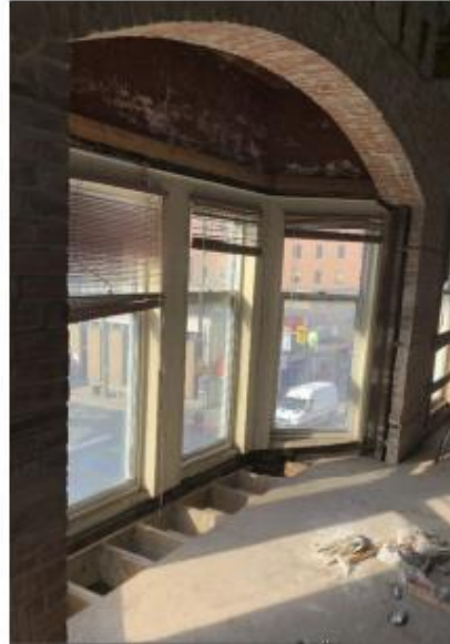
Figure 26: Detached base framing of the bay window on the second floor.
