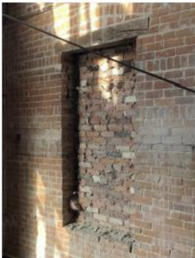
Figure 32: Infilled window on the second floor of the north façade.
