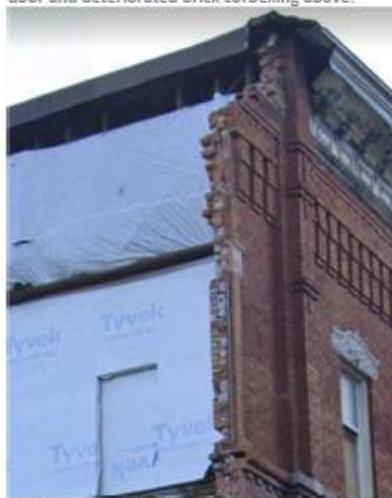
Figure 9: Exposed masonry at east end of north façade.
