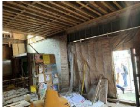
Figure 38: Openings on the ground level.
