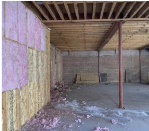
Figure 44: Interior condition of second floor walls.
