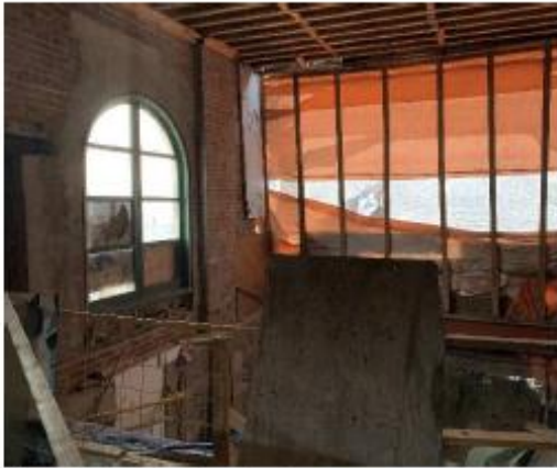
Figure 39: Interior of northeast corner.
