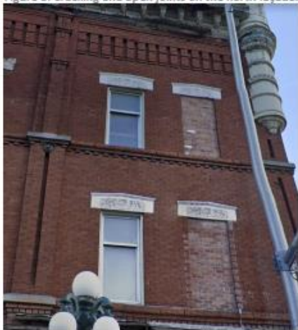
Figure 8: Cracking and open joints on the north façade.
