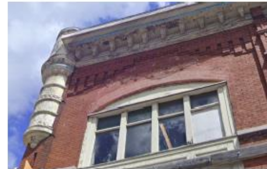
Figure 14: Deteriorated brick above previous location of bay windows on the west façade.
