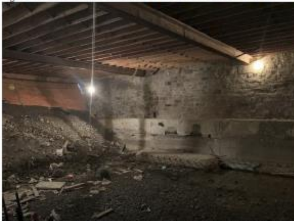
Figure 51: Backfilling at the previous east wall and voids in the south foundation wall.
