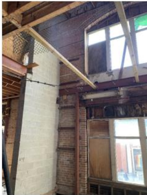
Figure 24: Interior of the large, fixed windows on the west façade.
