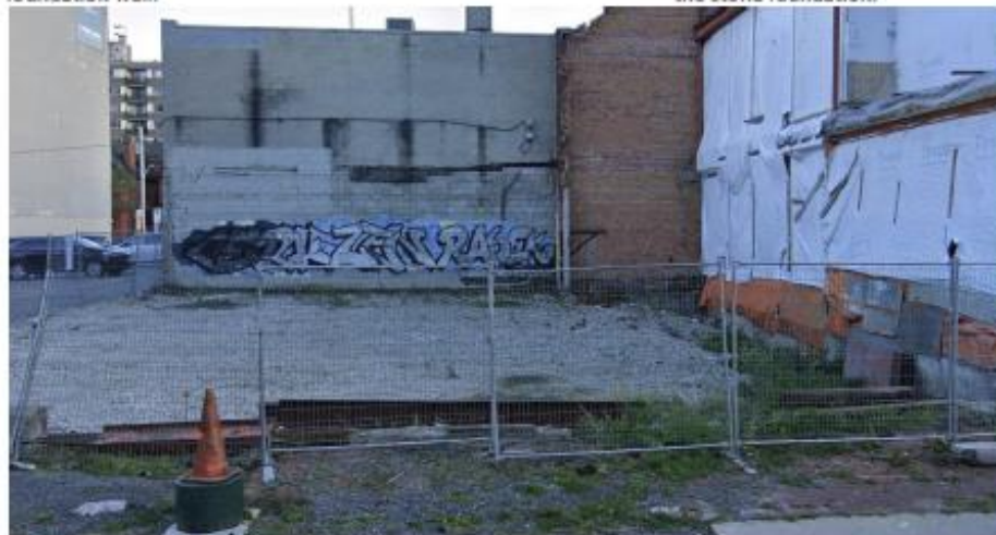
Figure 53: Backfilled location of previous addition, sloping towards the remainder of Somerset House.
