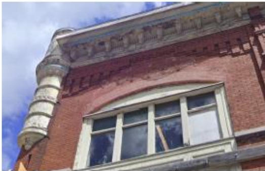
Figure 14: Deteriorated brick above previous location of bay windows on the west façade.
