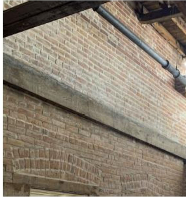
Figure 46: Deteriorated brick on interior of third floor with debonded wythes, frost damage, and surface damage.
