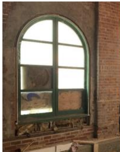
Figure 30: Interior of arched window on the north façade.
