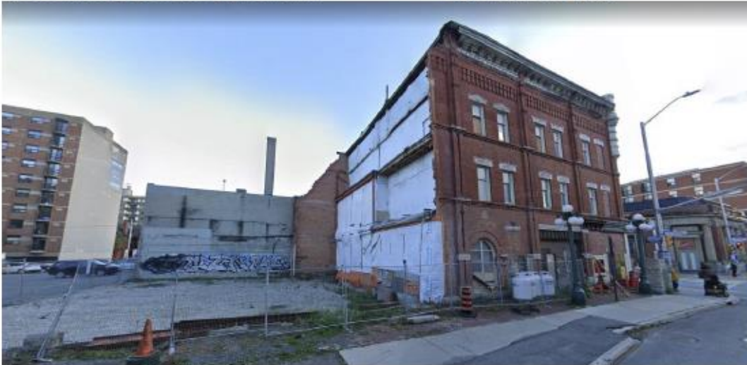
Figure 5: Current state of the building
