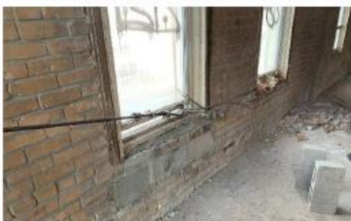
Figure 33: Interior of second floor windows on the north façade.
