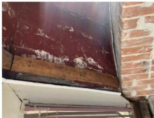
Figure 26: Detached base framing of the bay window on the second floor.
