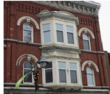
Existing Bay Window Structure to be Reconstructed
