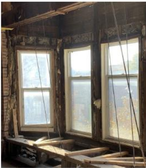
Figure 27: Interior side of the first floor bay window.
