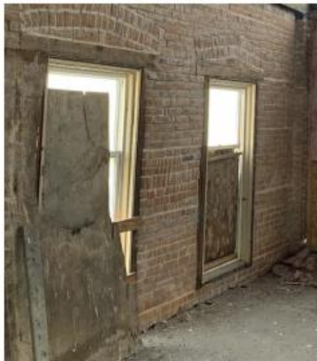
Figure 31: Interior of third floor windows on the north façade.
