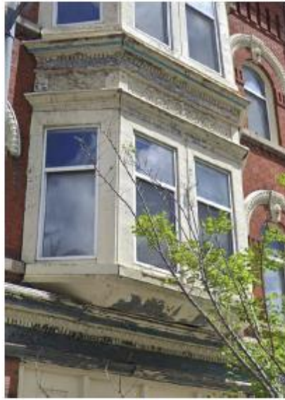
Figure 22: Exterior of the bay window on the west façade.
