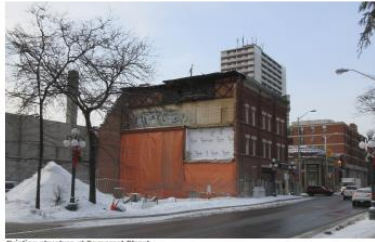
Existing structure at Somerset Street
