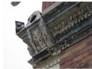
Cornice Brackets to be restored
