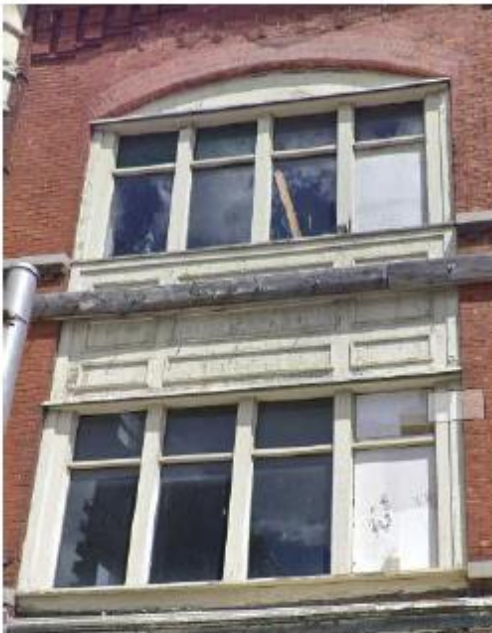
Figure 23: Exterior of the large, fixed windows on the west façade.
