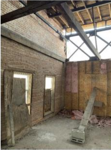
Figure 45: east wall supports on the third floor.
