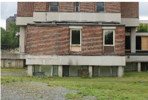
Photo 42: First storey of north façade, looking south
