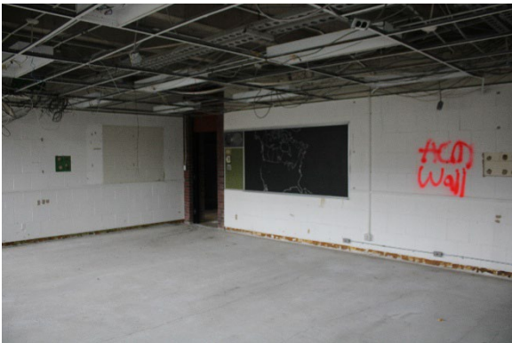
Photo 88: Representative second storey classroom
