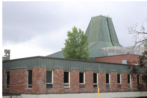
Photo 30: Rear (north) façade, looking southwest
