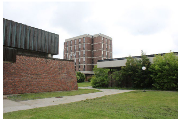
Photo 58: West façade, looking northeast
