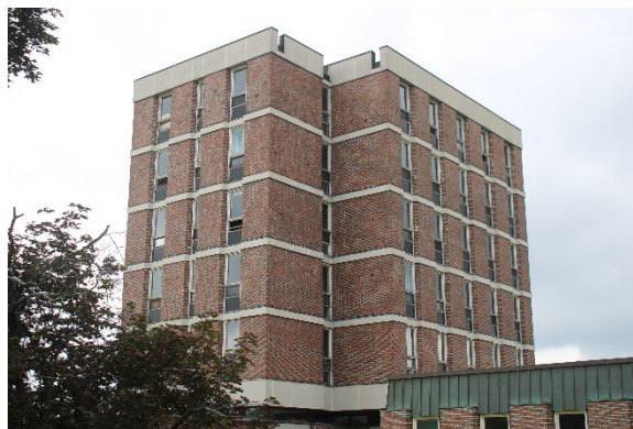
Photo 43: North and west façades, looking southeast
