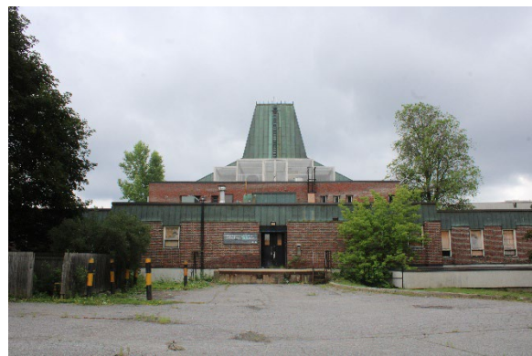
Photo 17: North façade of Building A, looking south
