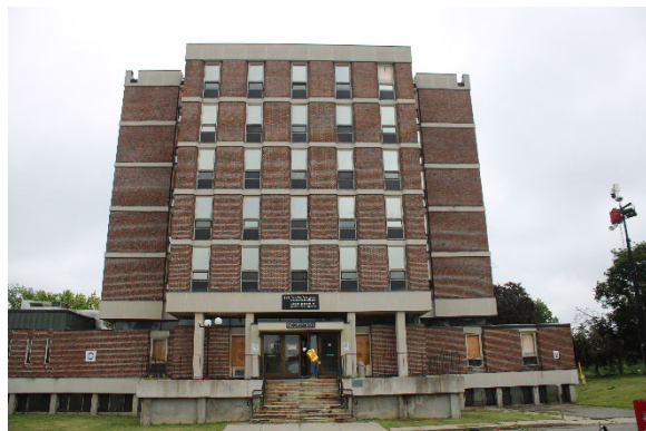
Photo 37: Front (east) façade, looking west
