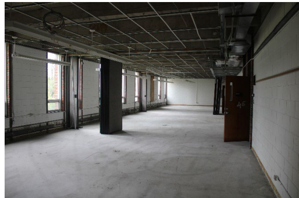
Photo 89: Representative third storey classroom
