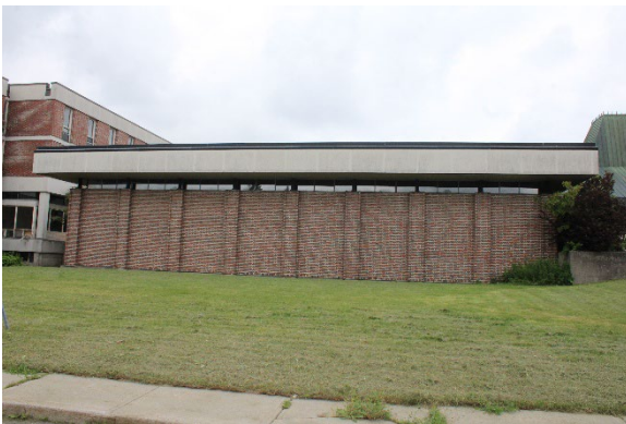
Photo 57: East façade, looking west
