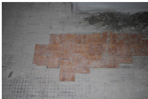
Photo 23: Concrete flooring and remaining parquet flooring
