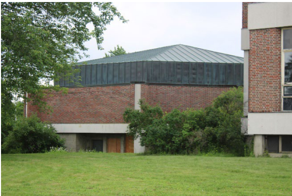
Photo 75: East façade, looking west
