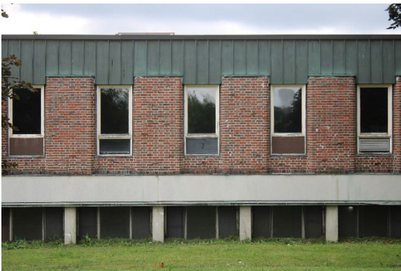
Photo 29: Rear (north) façade, looking south
