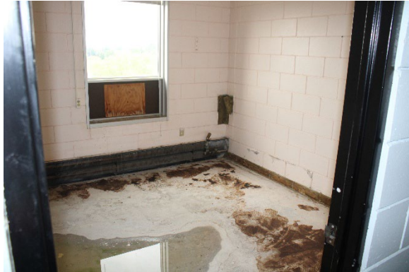
Photo 103: Representative sixth storey room
