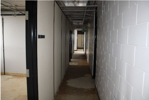
Photo 51: Representative fourth storey hallway
