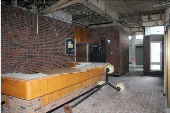
Photo 45: Former front foyer
