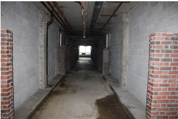
Photo 82: Representative first storey hallway
