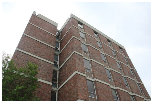
Photo 95: North façade, looking south
