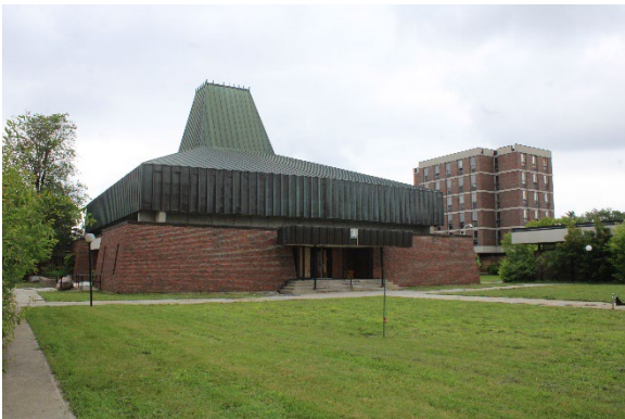
Photo 14: Building A, front (south) façade, looking northeast
