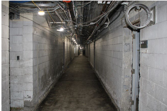
Photo 105: Representative basement hallway
