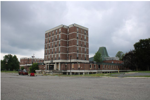
Photo 34: Building C, looking southwest
