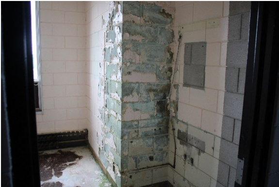
Photo 104: Representative sixth storey concrete walls
