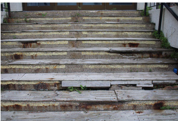
Photo 38: Front façade steps to entryway, looking west
