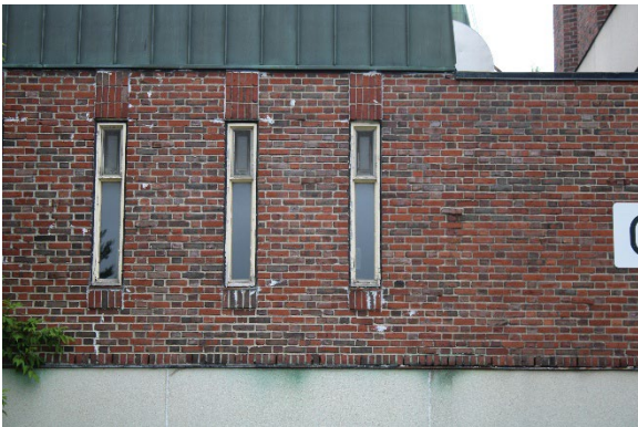
Photo 40: Front façade windows of south extension, looking west
