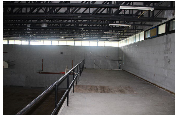
Photo 62: Mezzanine area in former gym
