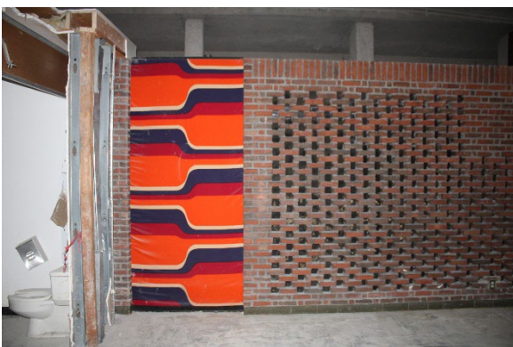
Photo 28: Brick wall around former altar area
