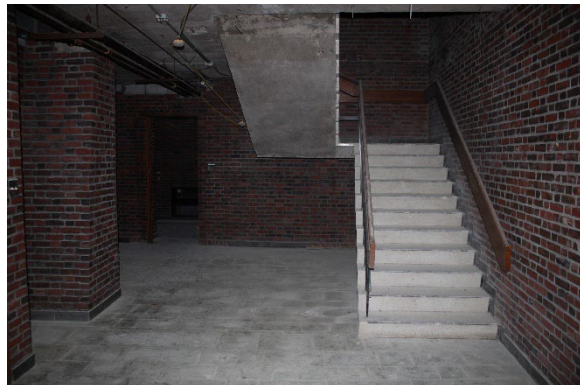
Photo 21: Interior stairs from basement to first storey
