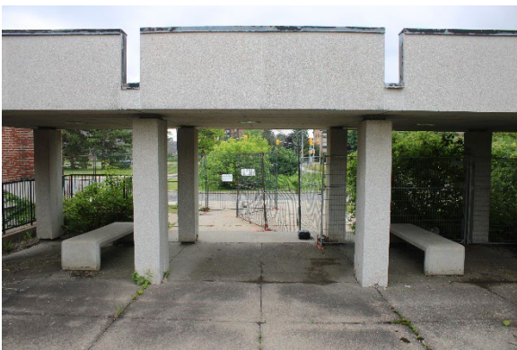
Photo 11: Concrete stairs up to academic courtyard, looking south
