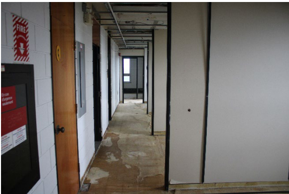
Photo 53: Representative fifth storey hallway
