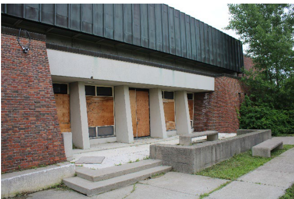
Photo 16: Front entrance to Building A, looking northeast
