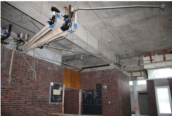
Photo 47: Interior poured concrete ceiling
