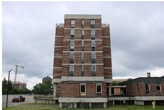
Photo 41: North façade, looking south
