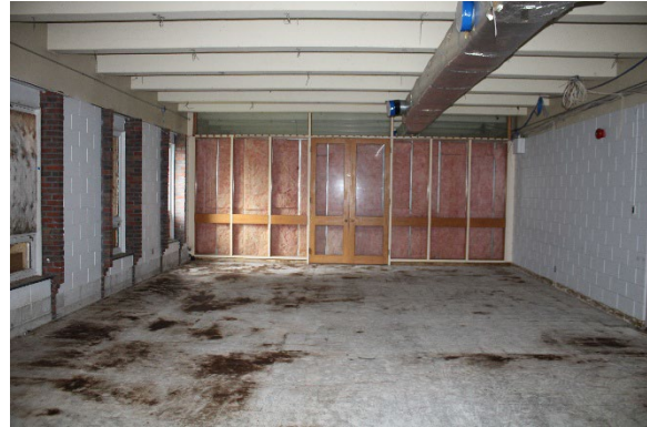
Photo 109: Representative classroom partition
