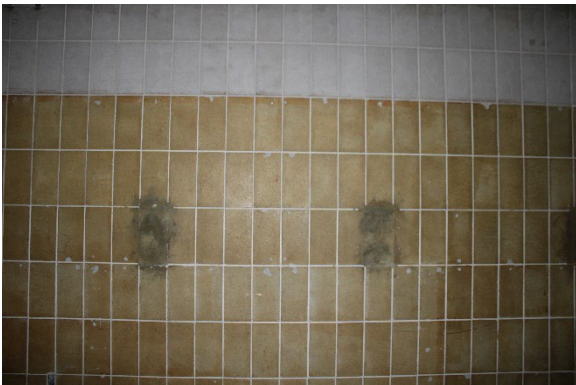
Photo 61: Representative wall cladding
