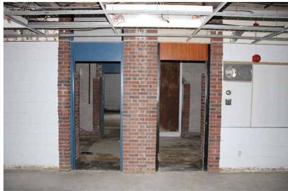
Photo 83: Representative first storey doorways
