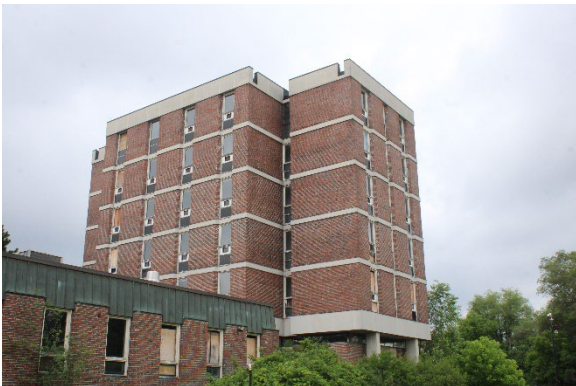
Photo 90: Building K, looking southwest
