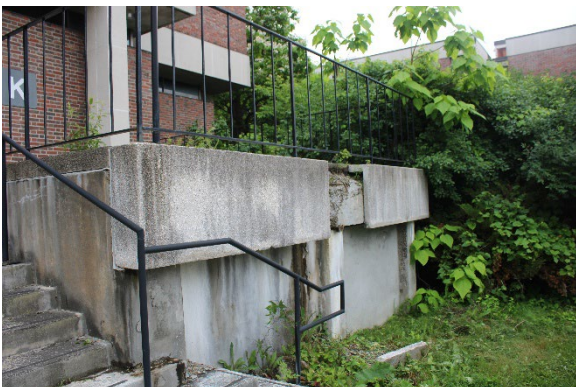
Photo 92: Raised concrete walkway, looking southeast
