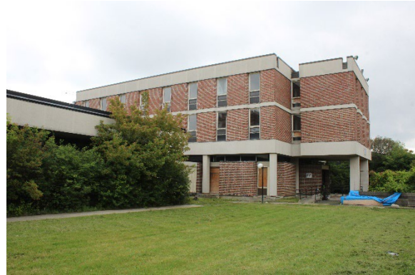
Photo 64: North façade, looking south east
