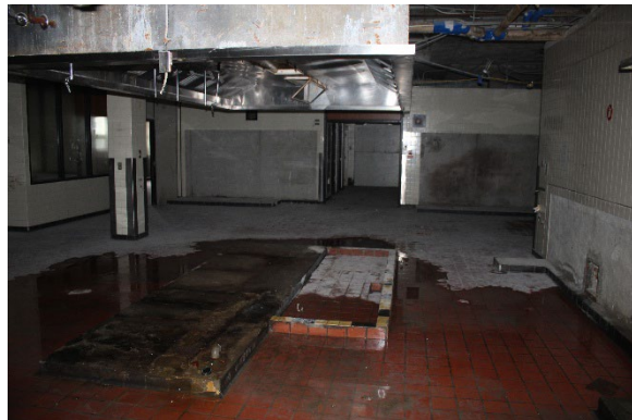
Photo 19: Former kitchen in basement
