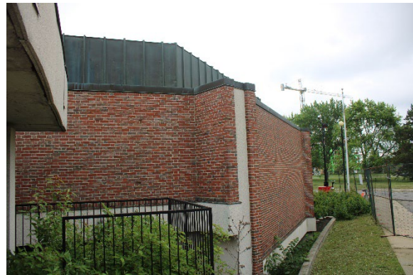
Photo 74: South façade, looking east
