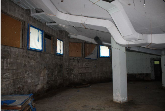
Photo 76: Basement space below theatre
