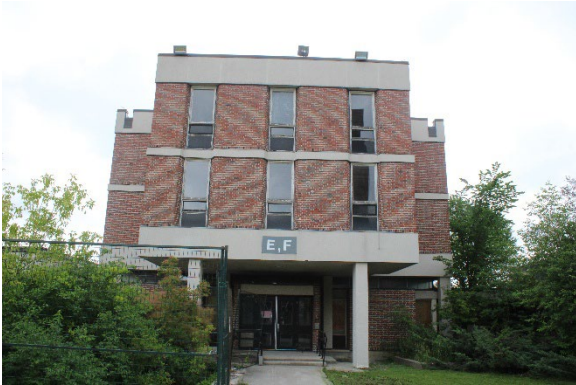
Photo 63: Front (west) façade, looking east
