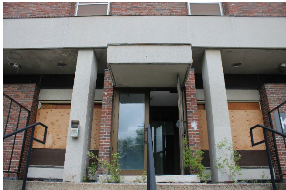
Photo 91: Front entryway, looking east
