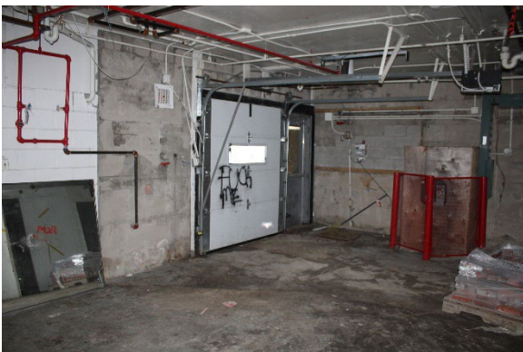
Photo 106: Representative basement room
