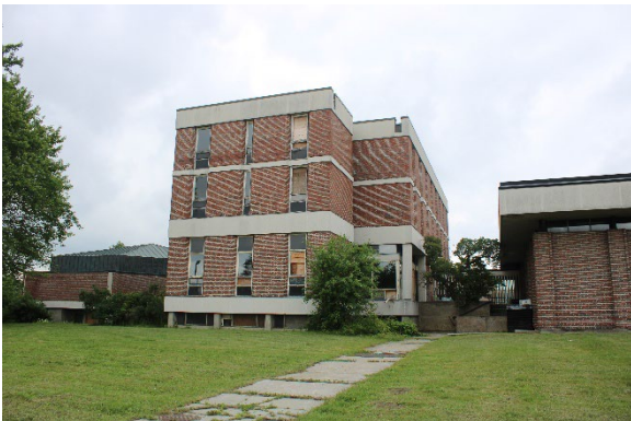
Photo 65: East façade, looking west
