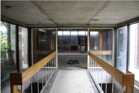
Photo 66: Hallway from Building F to Building E
