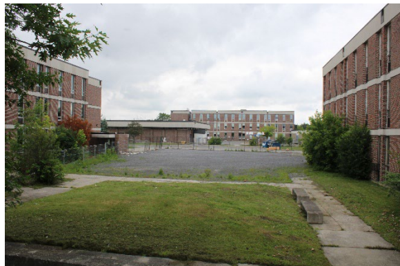
Photo 8: Former location of Buildings H and I, looking west
