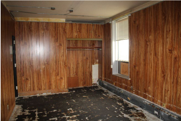
Photo 102: Representative second storey room
