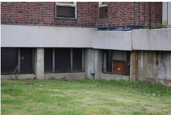
Photo 36: Foundation, looking west
