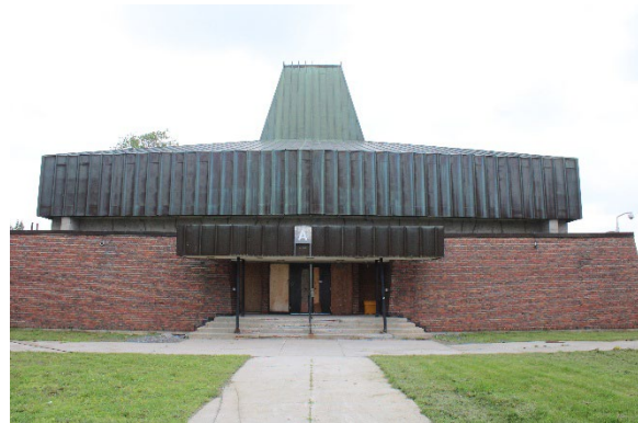
Photo 15: Building A, front (south) façade, looking north
