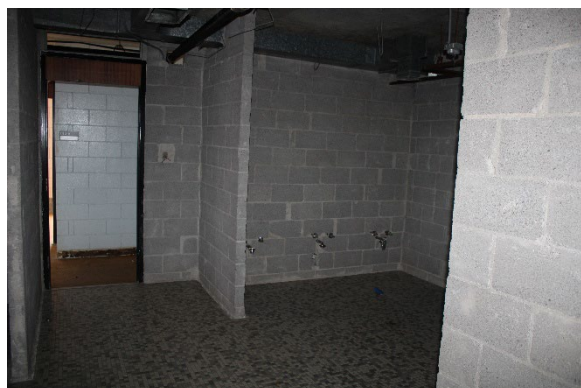
Photo 71: Representative communal bathroom, third storey
