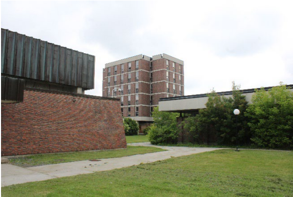
Photo 13: Academic courtyard, looking to Building C, looking northeast
