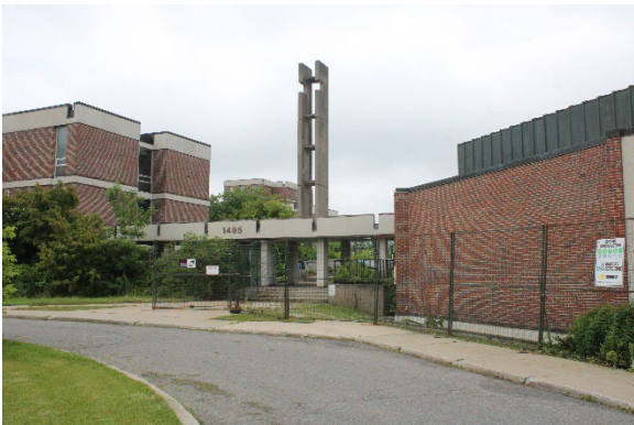
Photo 9: Entrance to academic courtyard from roundabout, looking north
