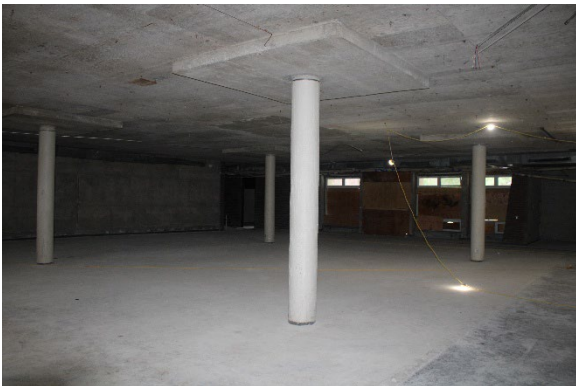
Photo 18: Former cafeteria in basement
