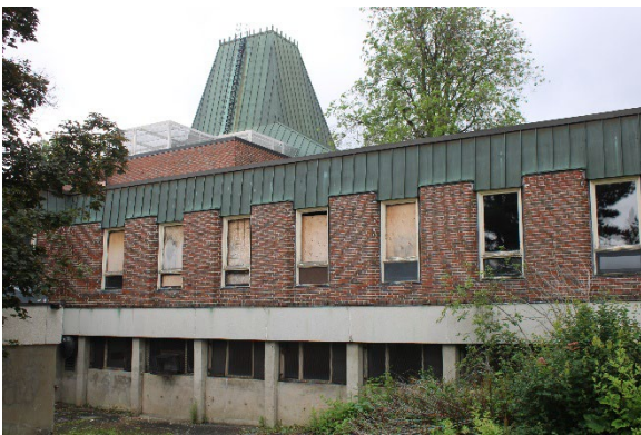
Photo 107: North façade, looking south
