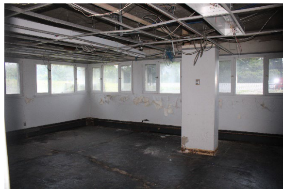
Photo 56: Representative basement room
