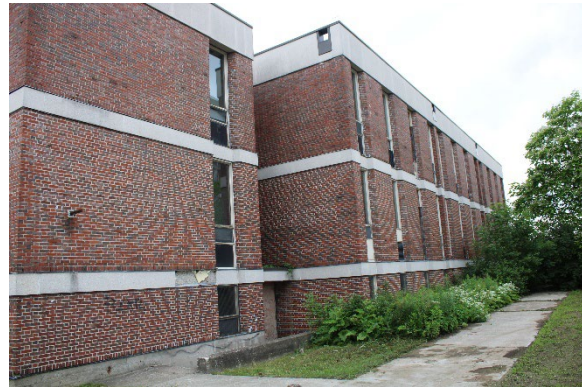
Photo 81: North façade, looking southwest
