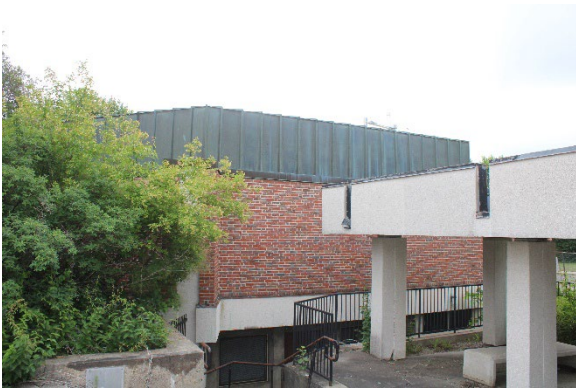
Photo 73: Southwest façade, looking east
