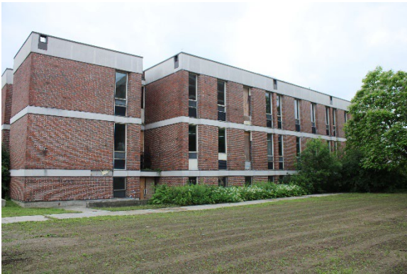
Photo 80: North façade, looking south
