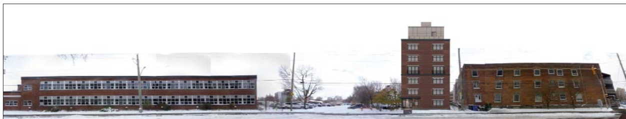
(Figure 14) 246 Gilmour Development - Streetscape View
