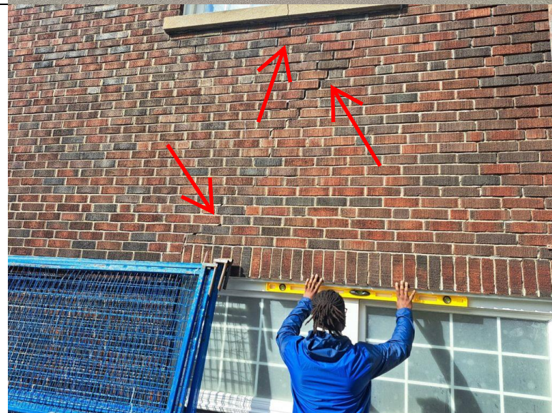
Photo 5 Stepped wide cracks noted along the South wall
