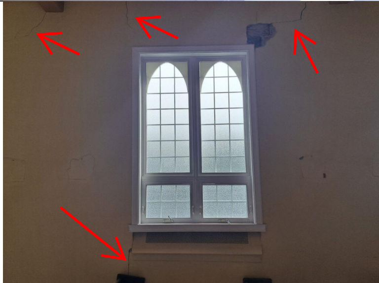
Photo 26 Cracks are noted along the left side (South) wall
