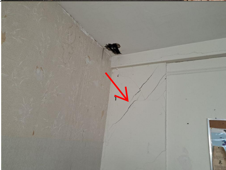
Photo 54 Diagonal cracks of the right (North side) wall
