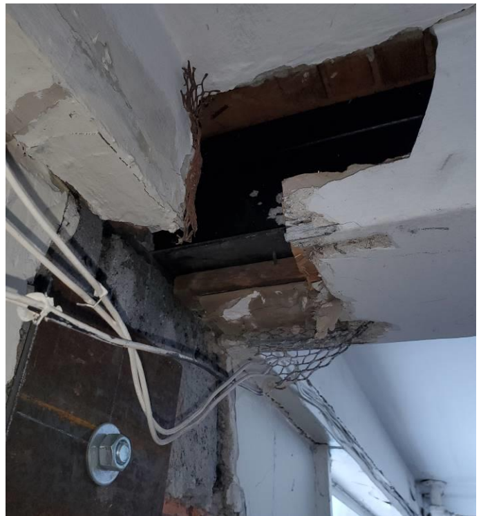
Figure 6: Steel Beam Sitting on Foundation Wall
