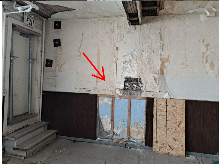
Photo 56 Horizontal crack of at least 5mm width at the rear side wall (East side) at the basement level
