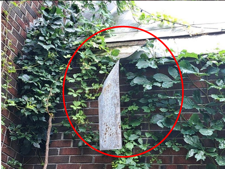
Photo 68 Flashing damage is noted
