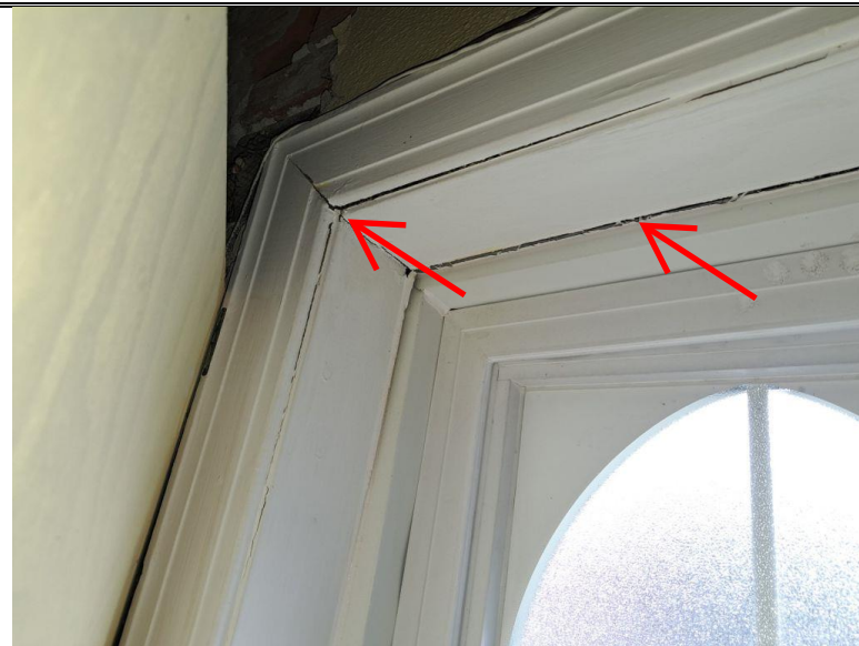
Photo 34 Sever damage and cracks to the fire exit door at the Southeast corner
