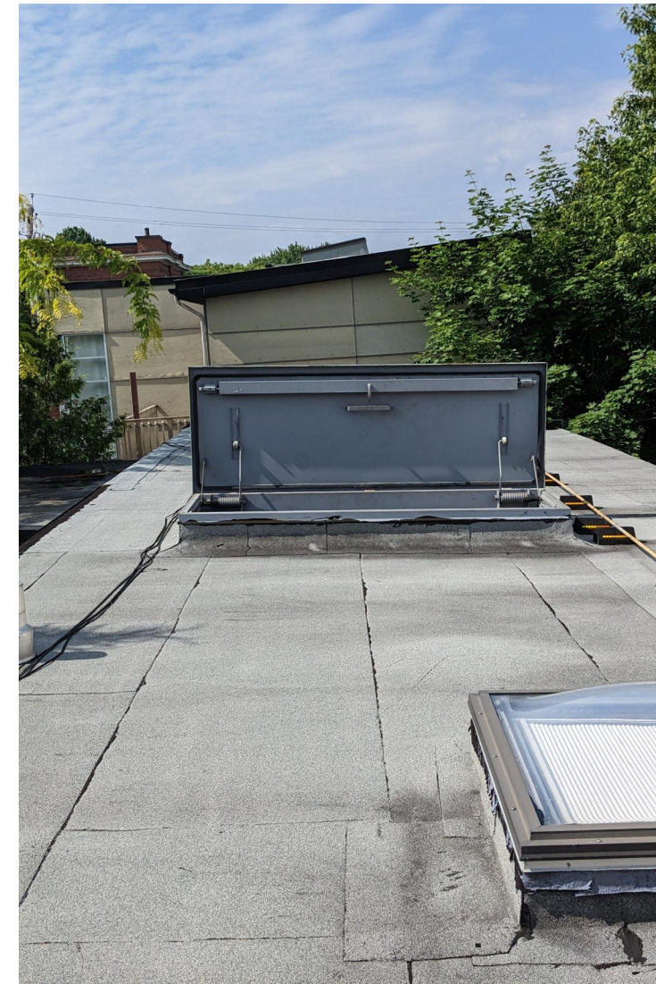
ROOFTOP VIEW (SOUTH)
