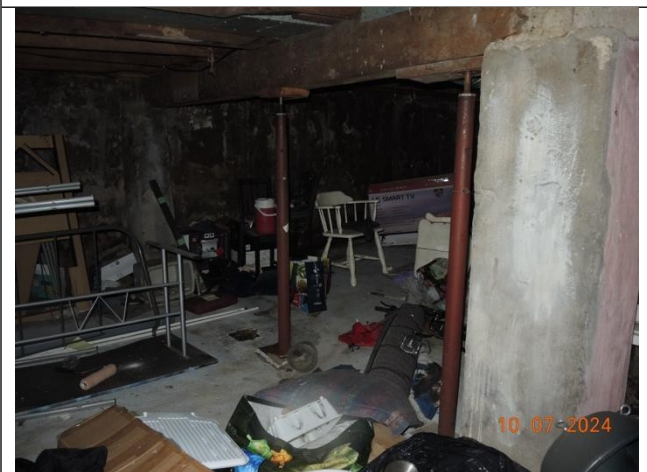
Photo 17: Jackposts and steel beam installed to support sagging floors.
