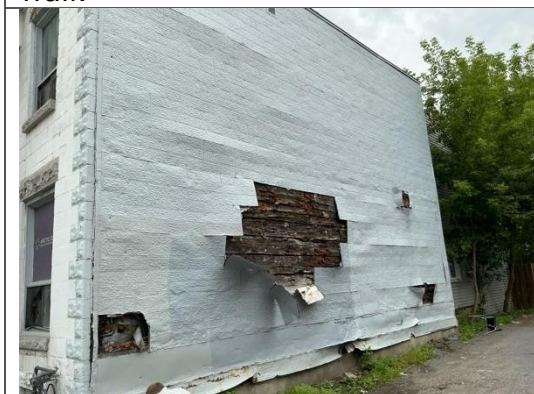
Photo 13: View of East wall.
