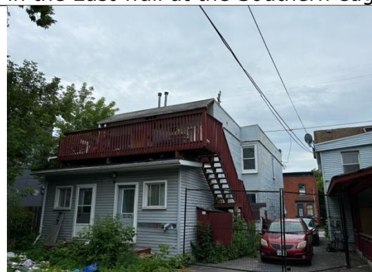
Photo 14: View of east wall and rear addition.
