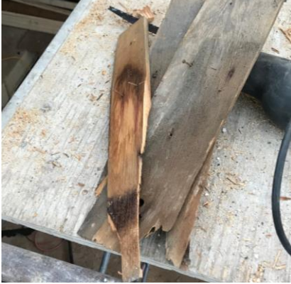
Figure 1-A: Record of roofing material. Source: Greg Statler documentation during construction.
