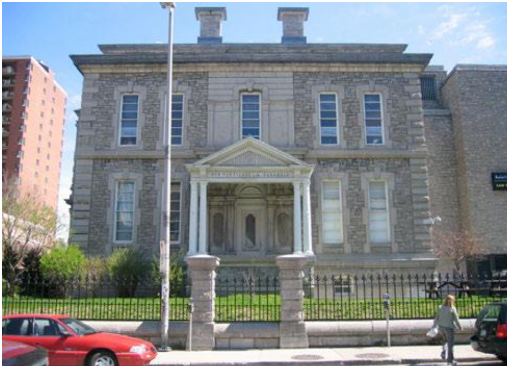
Figure 8: Carleton County Courthouse Nicholas Street façade. Note the masonry and metal perimeter wall/fence. The repositioned CRO has maintained the slit off axis interpretation. Source: B. Padolsky Associates Inc. 2013
