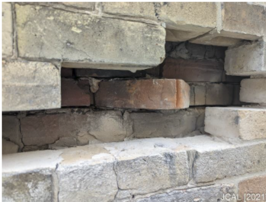
Photo 1g: Cavity and Diagonal Tying Brick [JCAL (2021)]
