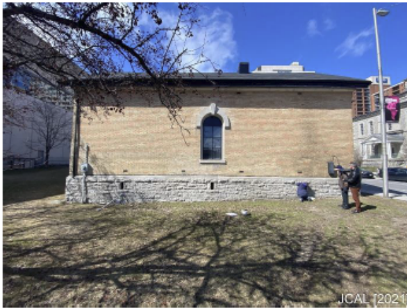
Photo 1c: South Elevation [JCAL (2021)]
