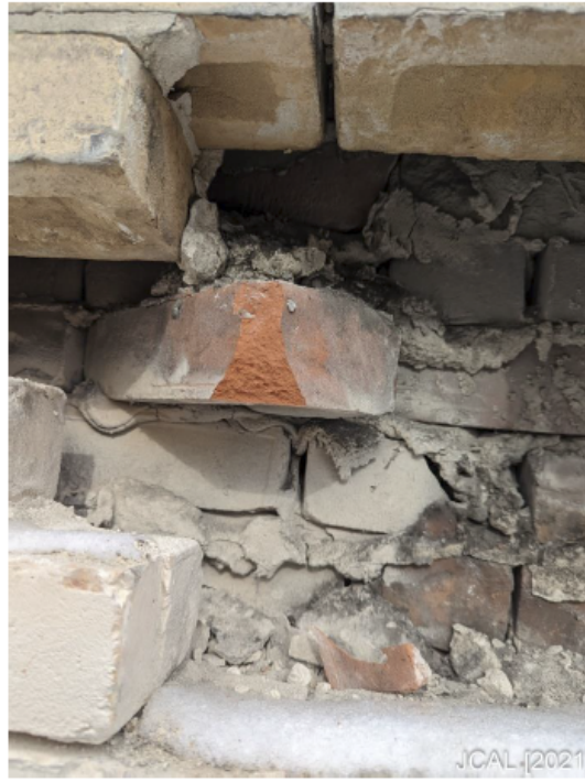
Photo 1f: Cavity and Diagonal Tying Brick [JCAL (2021)]
