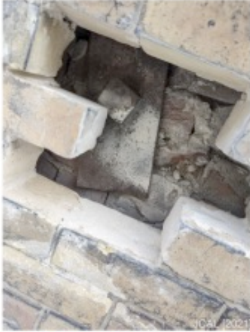
Photo 1i: Tie Rod End Plate [JCAL (2022)]
