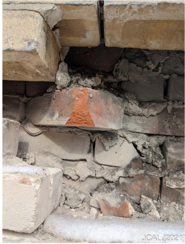
Photo 1f: Cavity and Diagonal Tying Brick [JCAL (2021)]
