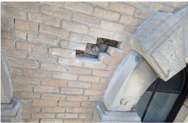
Photo 1k: Tie Rod End Plate [JCAL (2021)]
