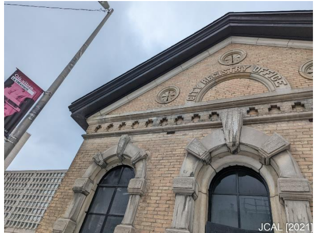
Photo 1b: Partial East Elevation [JCAL (2021)]
