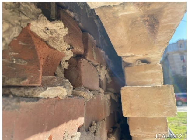
Photo 1d: Facing Brick and Cavity [JCAL (2021)]
