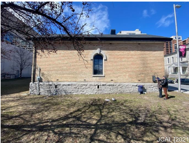
Photo 1c: South Elevation [JCAL (2021)]
