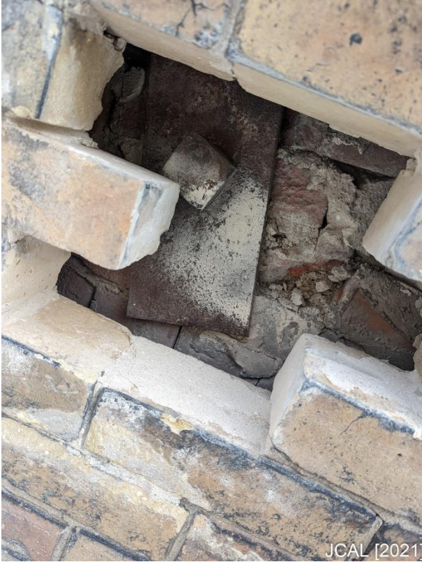
Photo 1i: Tie Rod End Plate [JCAL (2022)]
