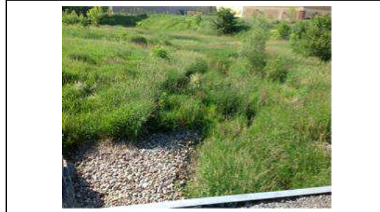
Location: Downstream Face Direction: Facing East
