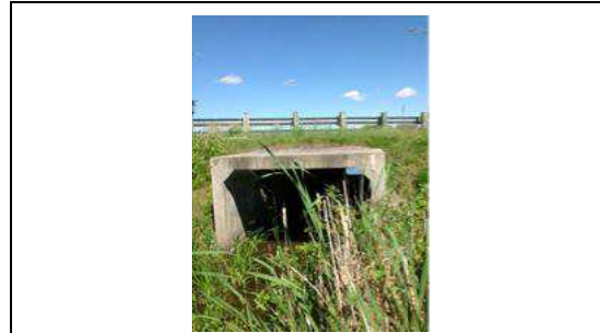
Location: Upstream Face Direction: Facing East
