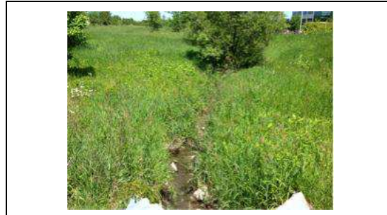
Location: Downstream Face Direction: Facing East
