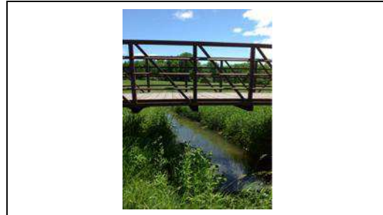
Location: Downstream Face Direction: Facing South
