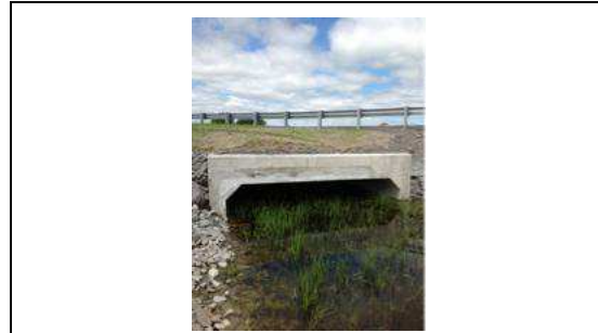
Location: Downstream Face Direction: Facing North
