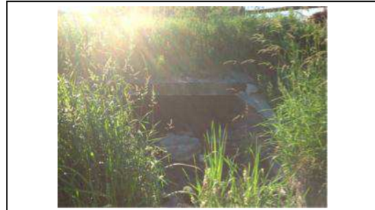
Location: Downstream Face Direction: Facing South
