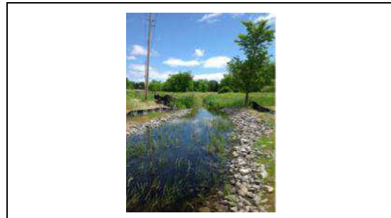
Location: Downstream Face Direction: Facing South
