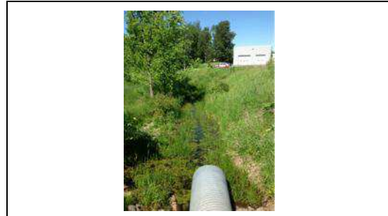
Location: Downstream Face Direction: Facing East
