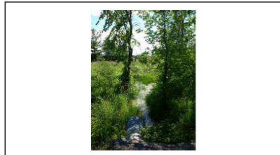
Location: Upstream Face Direction: Facing West
