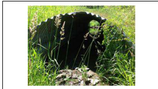
Location: Upstream Face Direction: Facing West
