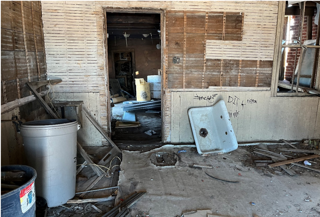
Photograph 3: First floor interior of the farmhouse.
