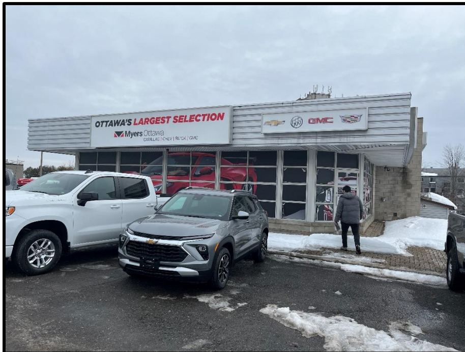
Photograph 6: View of the office/storage building in the southwest portion of the site.
