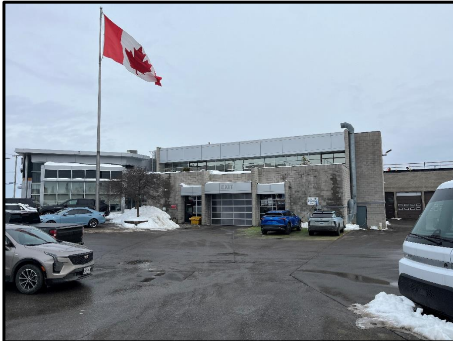
Photograph 7: View of the eastern elevation of the dealership building .
