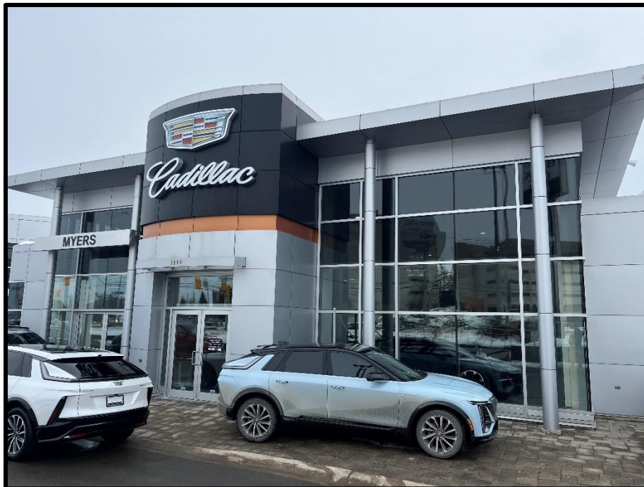
Photograph 8: View of the northern elevation and main entrance of the dealership building .
