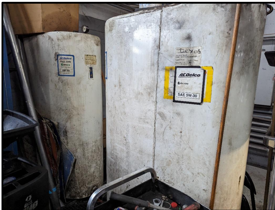
Photograph 16: View of the 2x motor oil ASTs in the northwest corner of the service bays.
