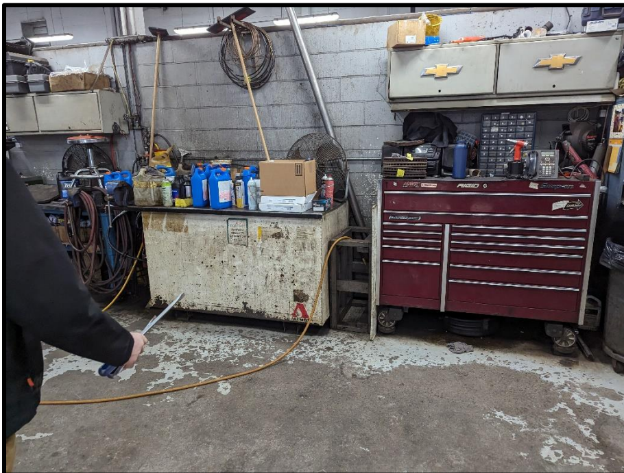
Photograph 12: View of the eastern bench style motor oil AST.
