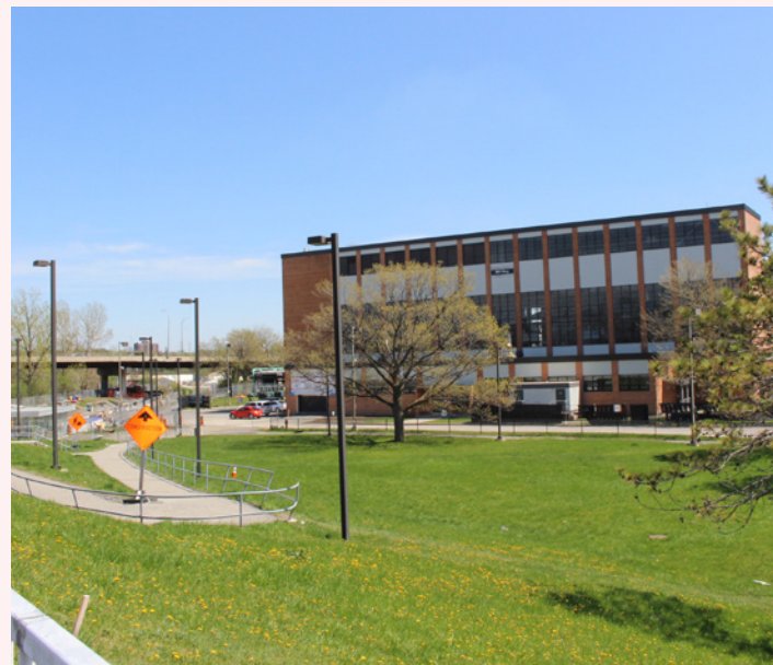
Figure 121: Existing conditions near the CHCP. Source: Fotern
