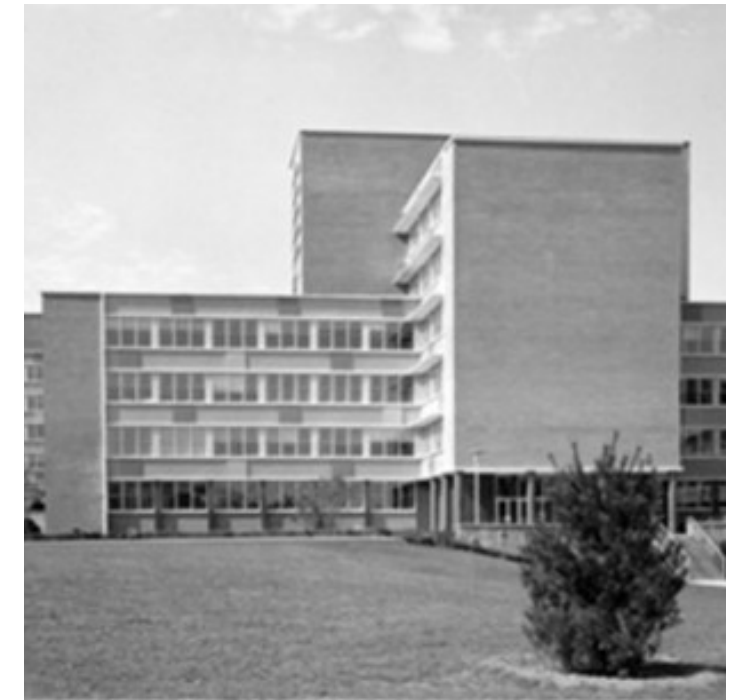
Figure 85: Sir Charles Tupper Building. Source: CLC
