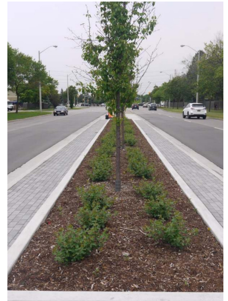
Figure 125: Stormwater tree trenches in Mississauga, ON. Source: CVC
