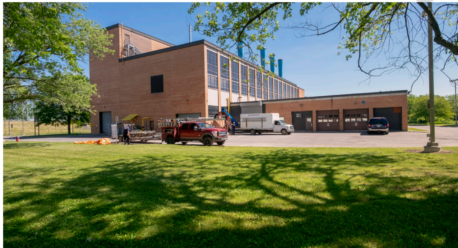
Figure 111: Central Heating and Cooling Plant Building. Source: CLC
