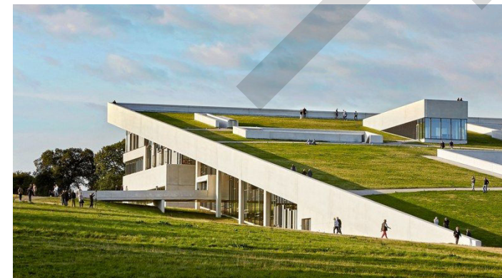
Figure 127: Green roof. Source: Henning Larsen Architects
