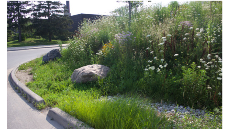
Figure 124: Bioswale. Source: Fotenn
