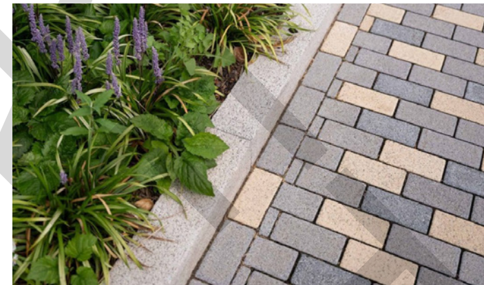
Figure 126: Permeable paving. Source: Fotenn
