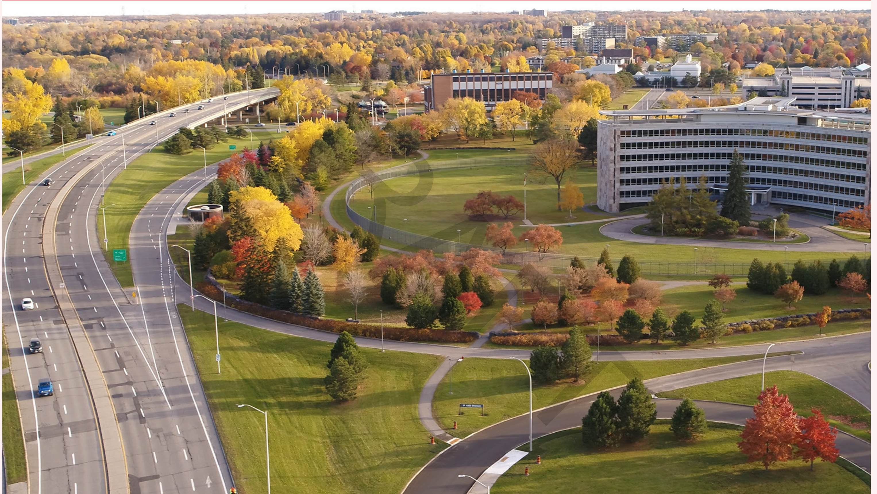
Figure 31: Bronson Ave and ramps. Source: CLC
