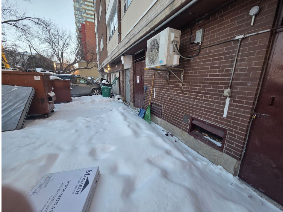
Photograph 7: View hydro Ottawa room on the ground floor of the residential apartment at 131 Parkdale Avenue, view is looking south.
