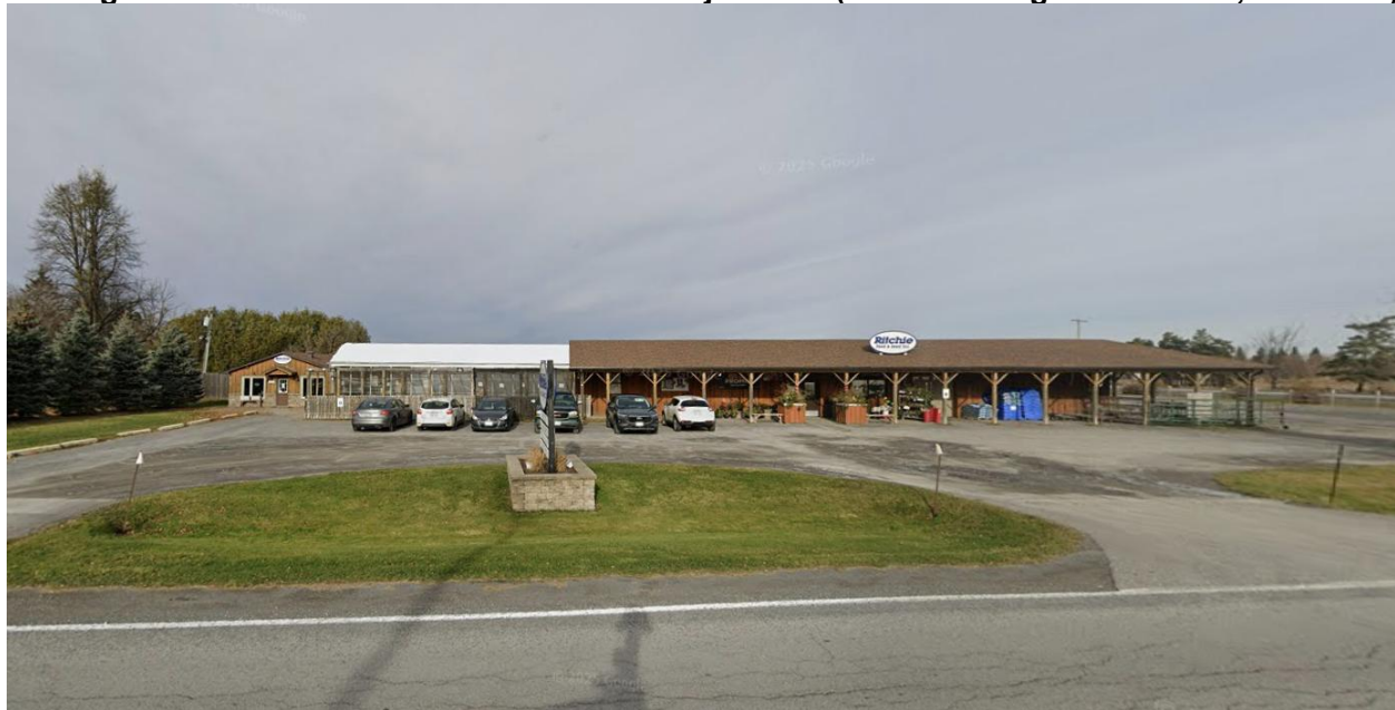
Figure 4: Land uses to the north of the Subject Site (Source: Google Streetview, Nov 2024)
