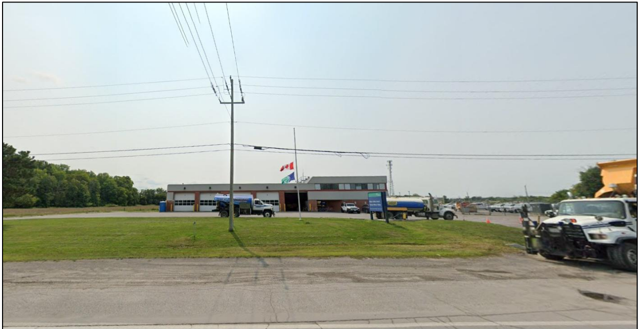
Figure 2: The municipal works and storage yard at 4244 Rideau Valley Drive abutting the Subject Site to the north looking west (Google Streetview 2021).
