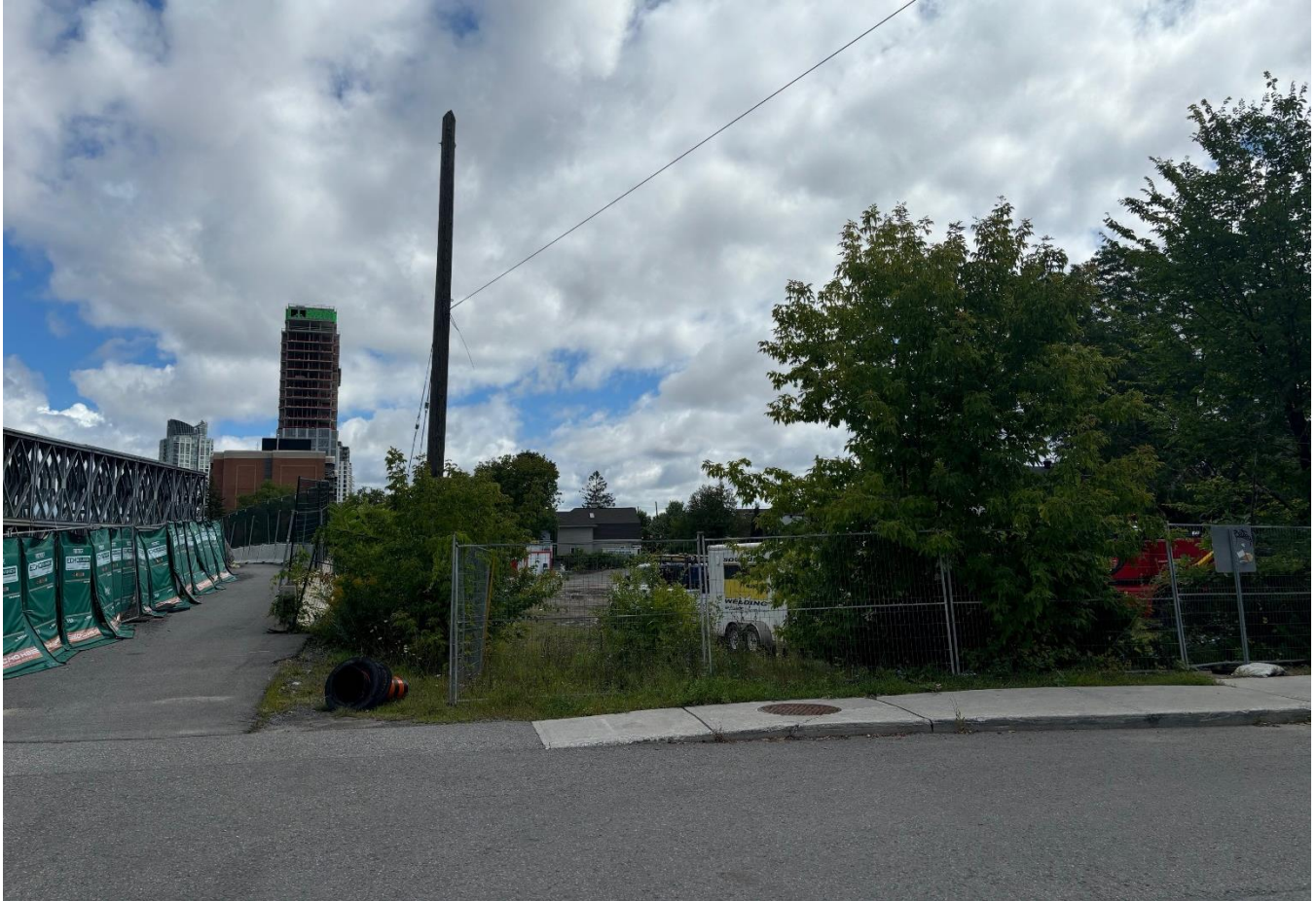
Figure 2: View of the subject property and MUP, looking northeast from Roosevelt Avenue. (Source: Fotenn Planning + Design, dated August 2024)
