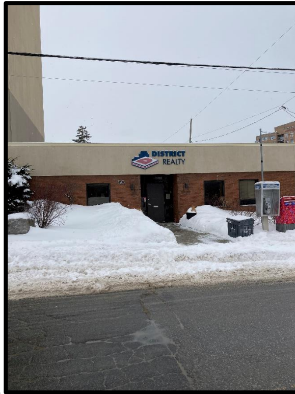
Photograph 1: View of the front of the 50 Bayswater Avenue office building, facing west.
