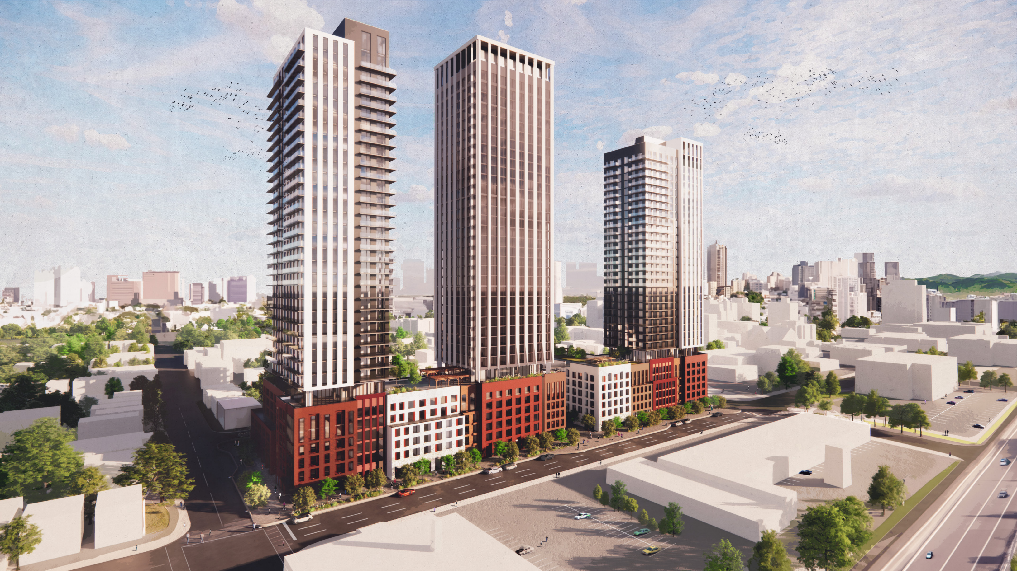
Updated View Looking Northeast Along Catherine Street
