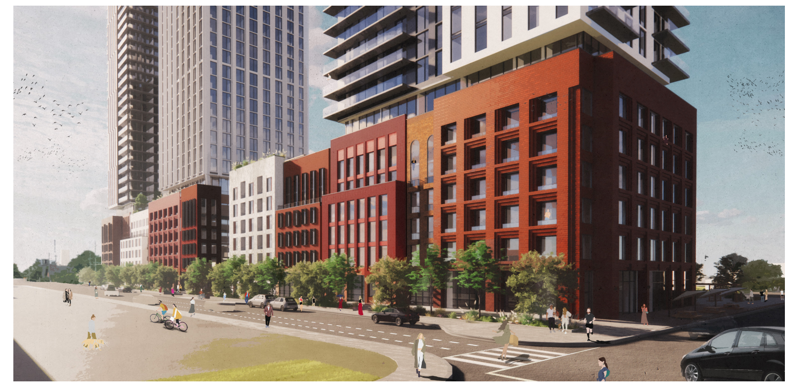
View Looking Northwest Along Cathrine Street
